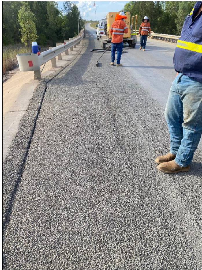
Figure 3: Spill location after clean-up works were completed.
