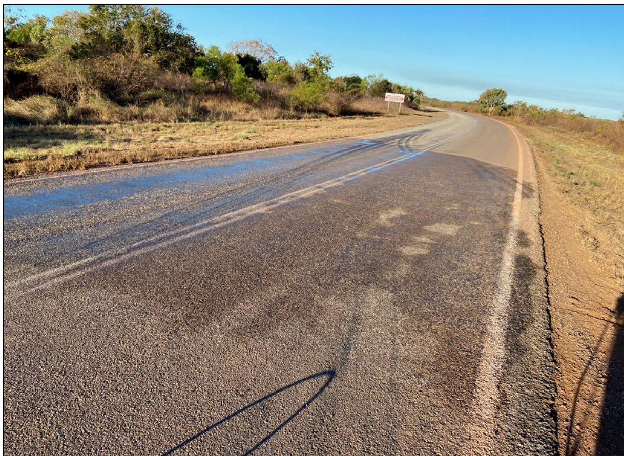
Image 3: During clean-up activities, a high-pressure hose was used to remove residual concentrate from the highway.
