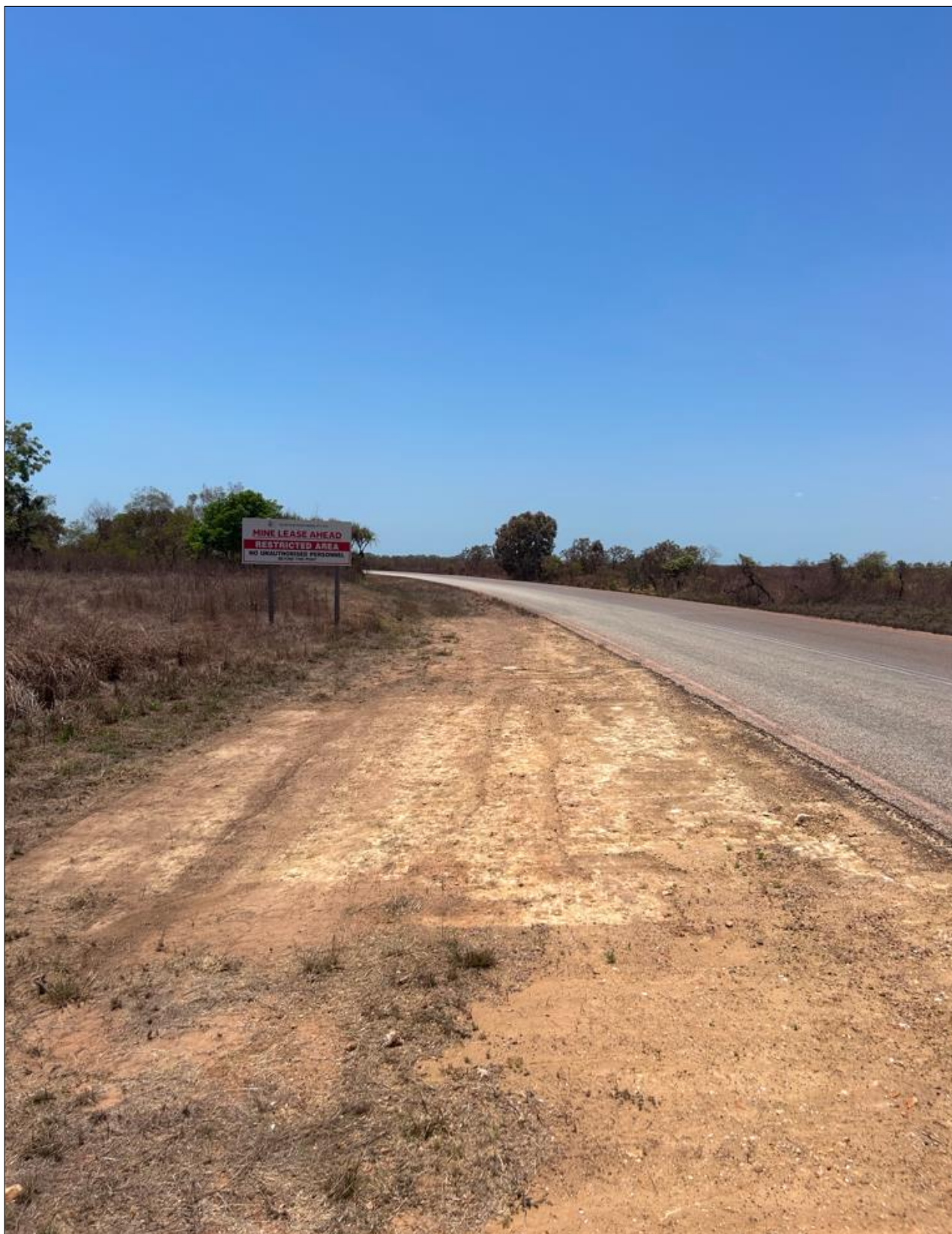
Image 5: Additional remediation works 10 October 2023; a bobcat was again used to remove potentially impacted surface material from the roadside adjoining the incident location.
