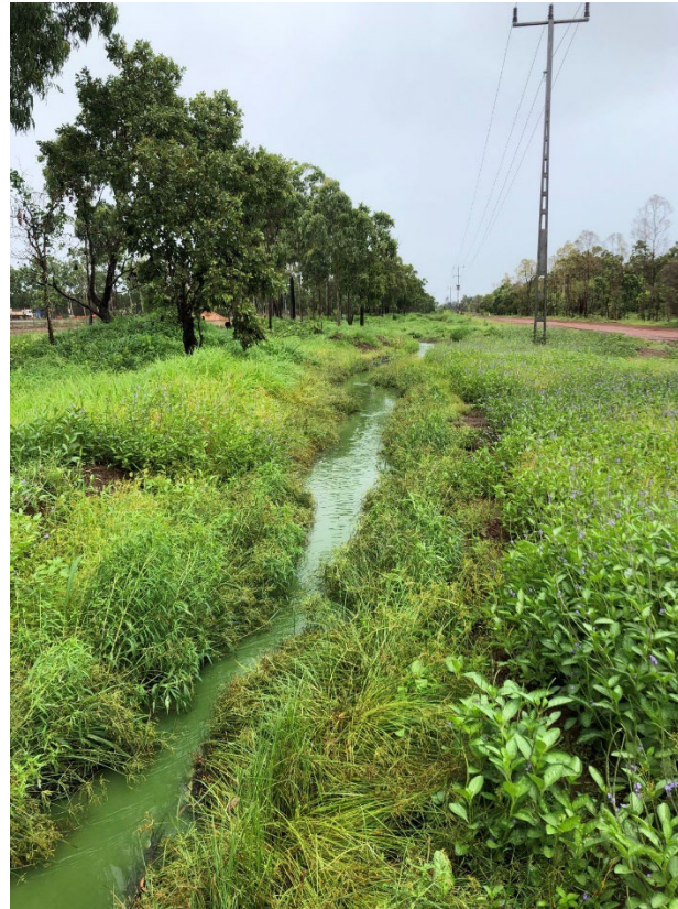
2. Northern boundary drain
