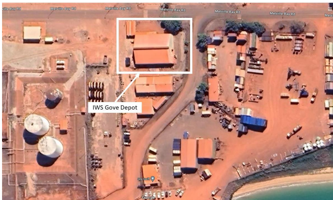
Figure 1 Cleanaway site overview
