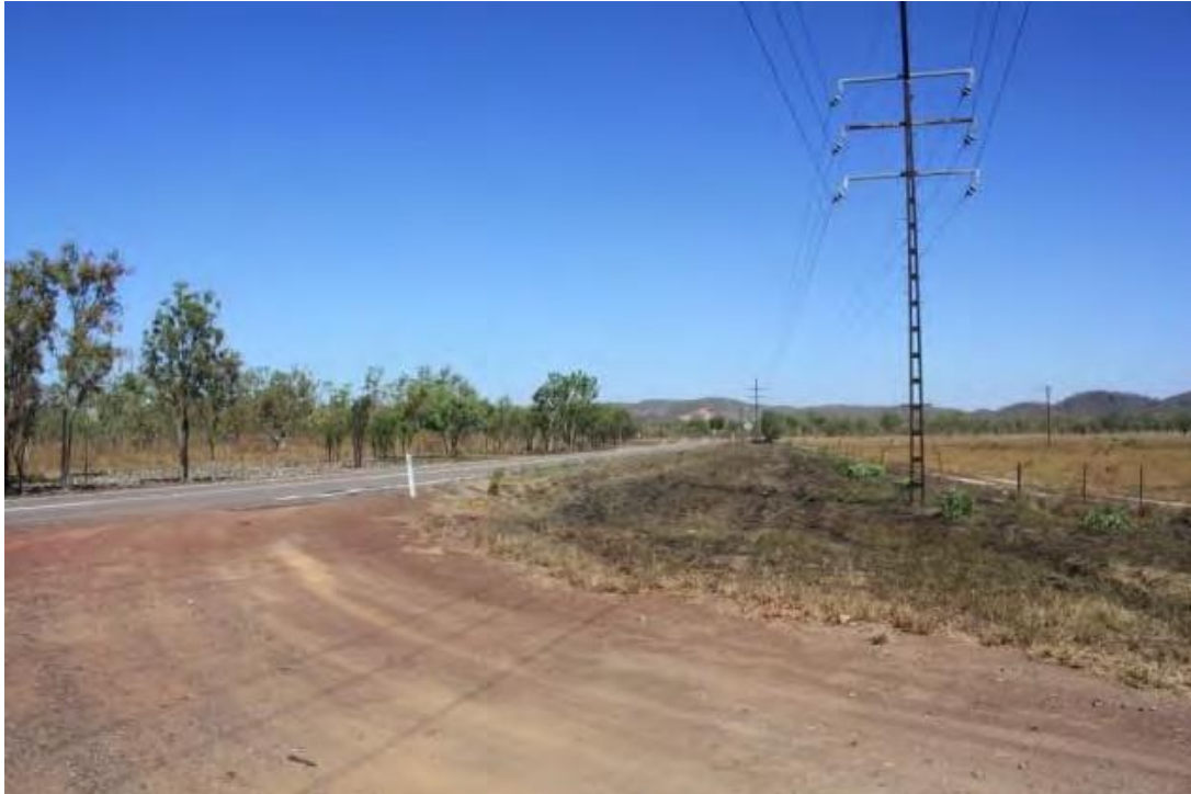
Figure 3: Site entrance West side of Arnhem Highway looking South
