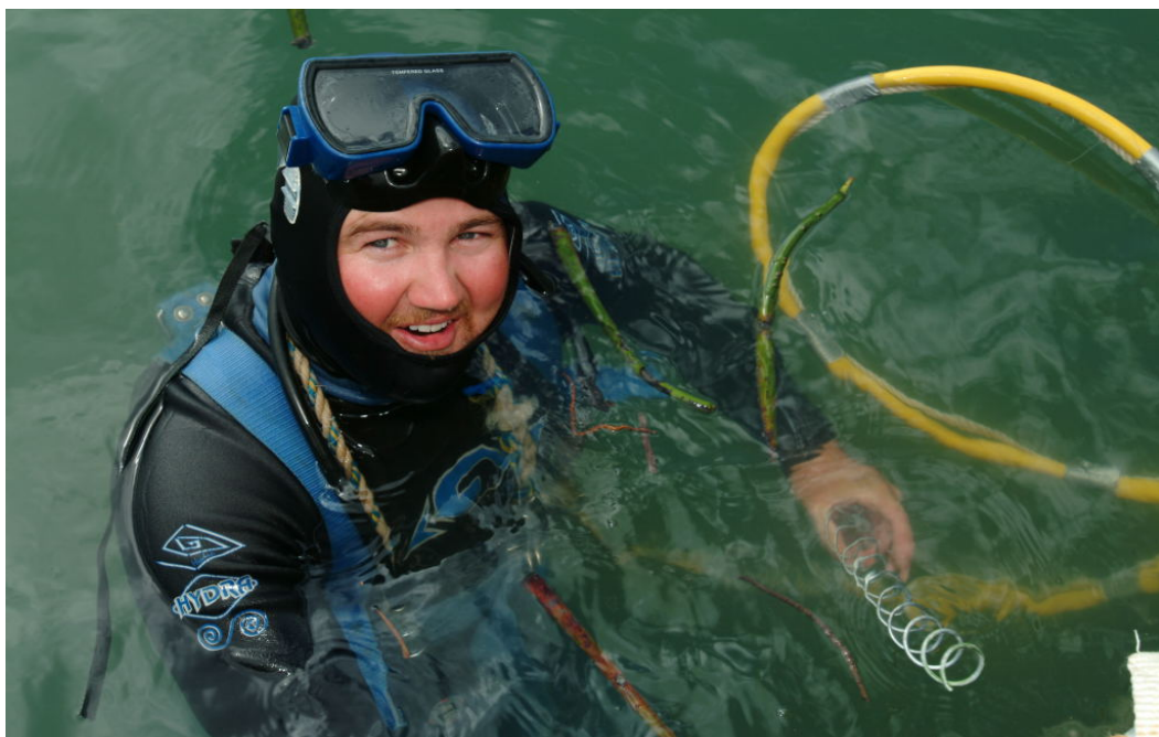
Plate 2: Diver Carrying Out Repairs on Port Hurd Farm Nets
