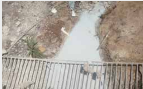
Polluted stormwater in watercourse
