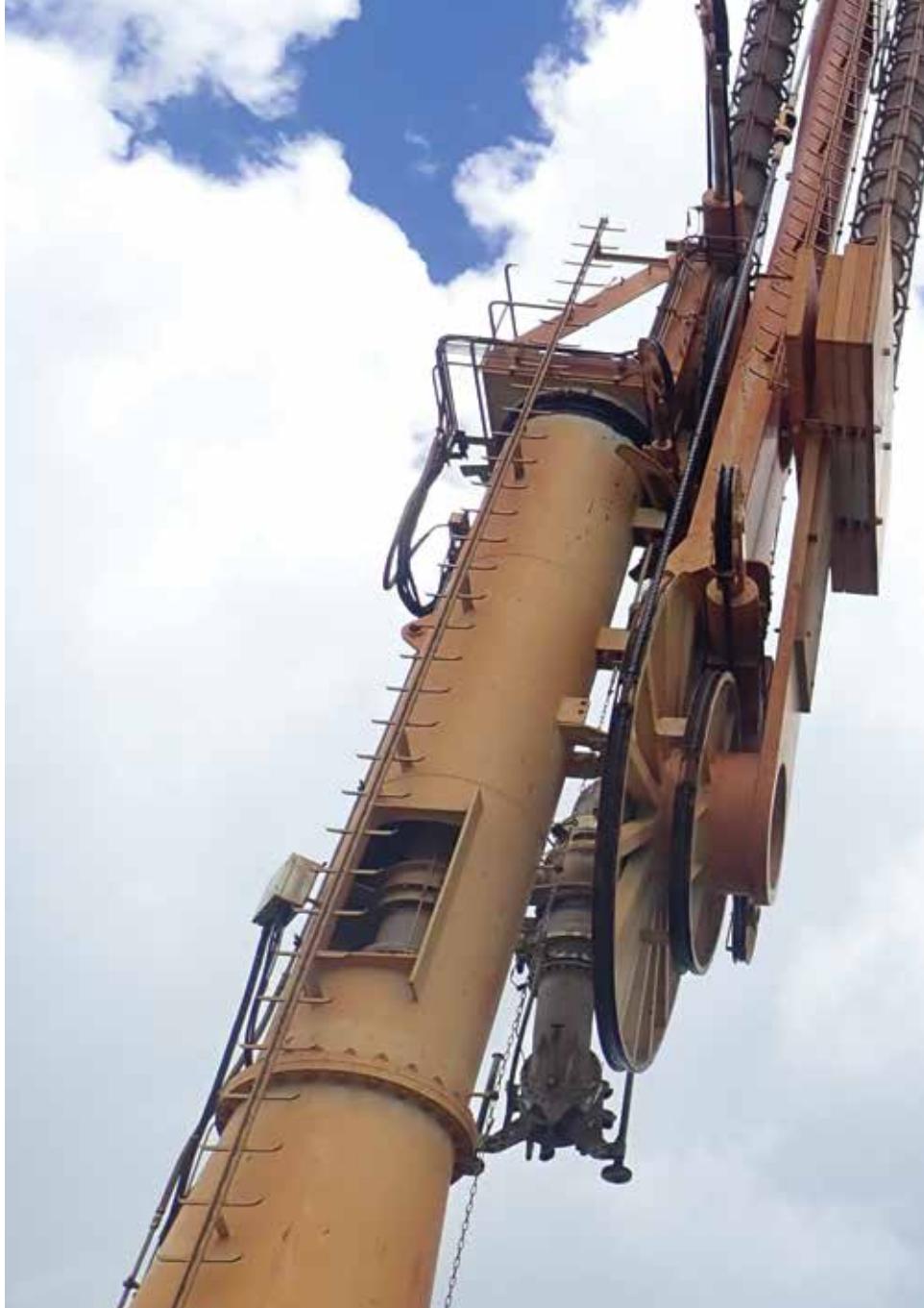
Photo: Shipping loading infrastructure
