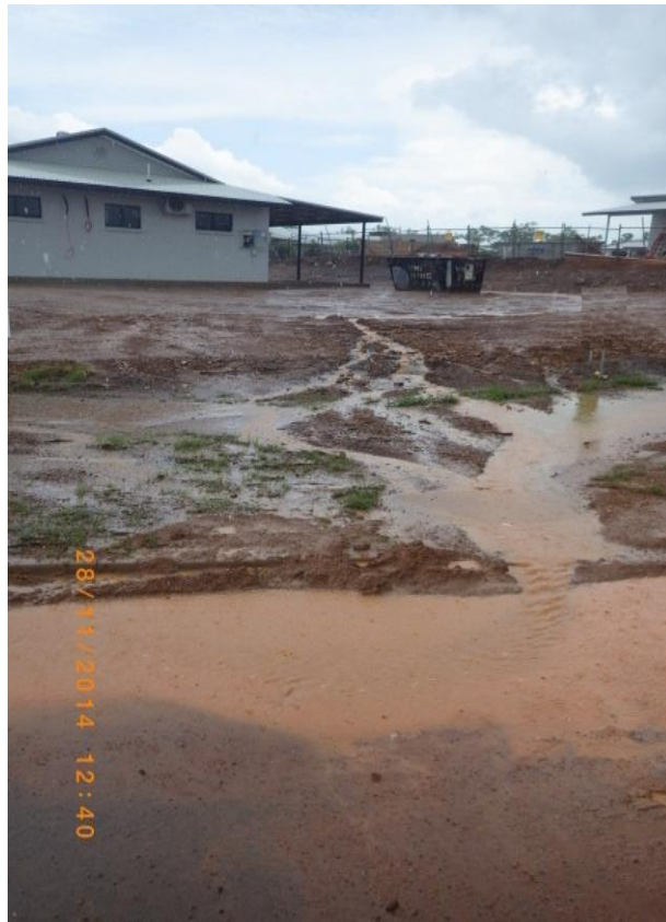
Figure 6-8: Overland discharge of muddy water onto road– no controls (NT EPA 2014)
