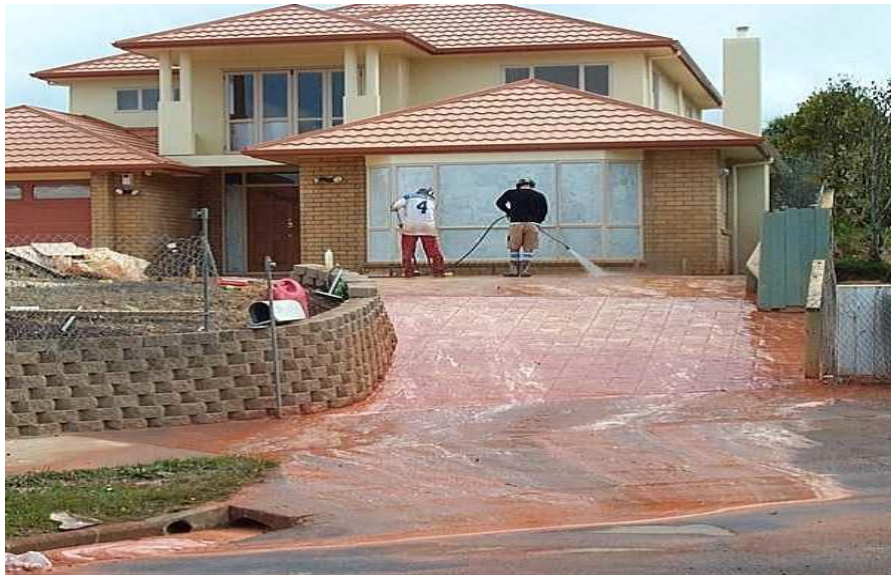
Figure 7-2: Washing of tile waste water discharging off site and into the stormwater (Source unknown)
