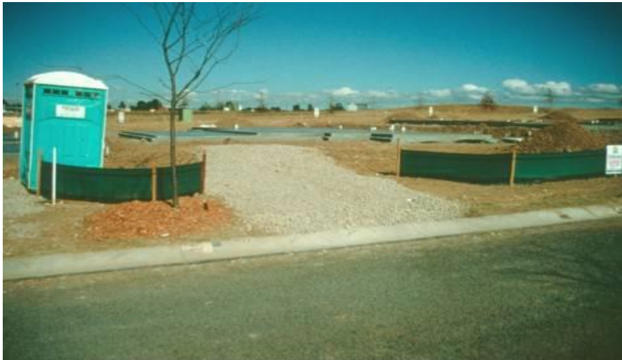
Figure 6-4: Another example of proper stabilised entry point (Environment Canterbury Regional Council)
