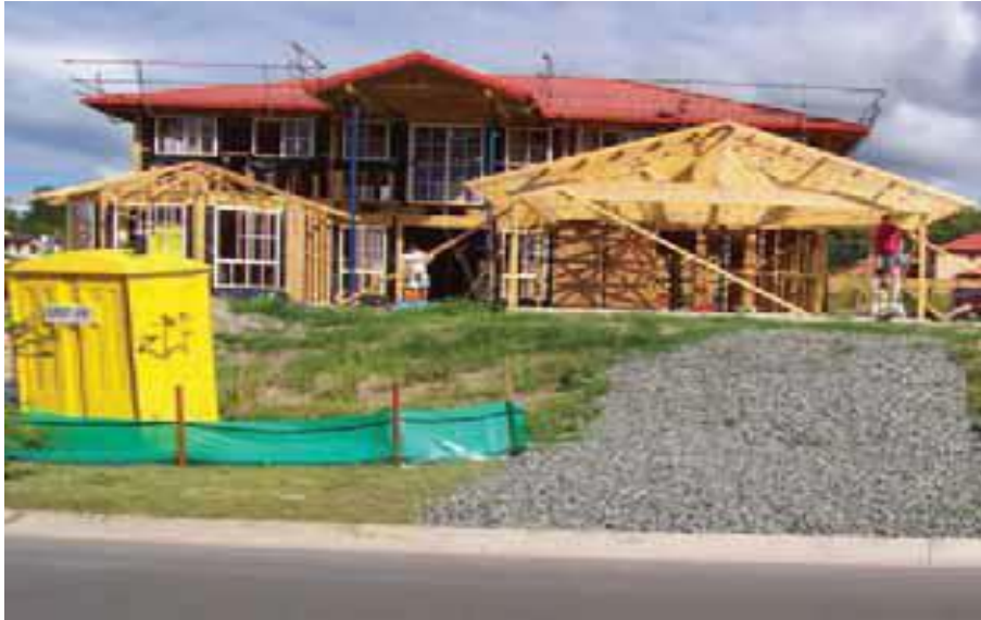
Figure 6-3: Properly stabilised entry point with nearby silt fence (Brisbane City Council)
