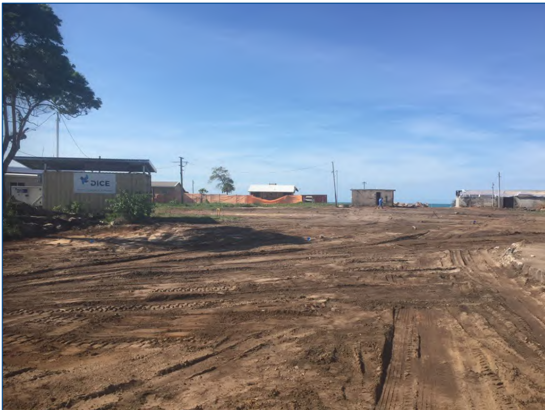
Final site condition looking north across central site area (22/11/2018)
