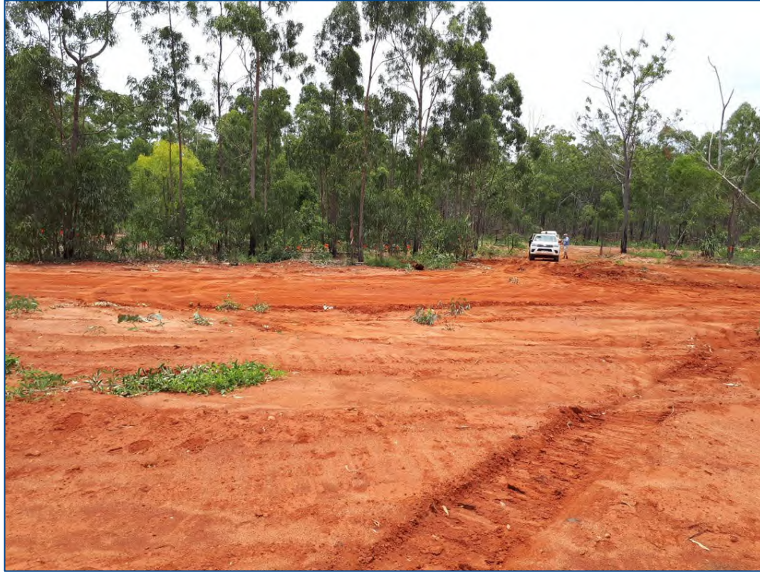
Final condition of containment cell (7/02/2019)
