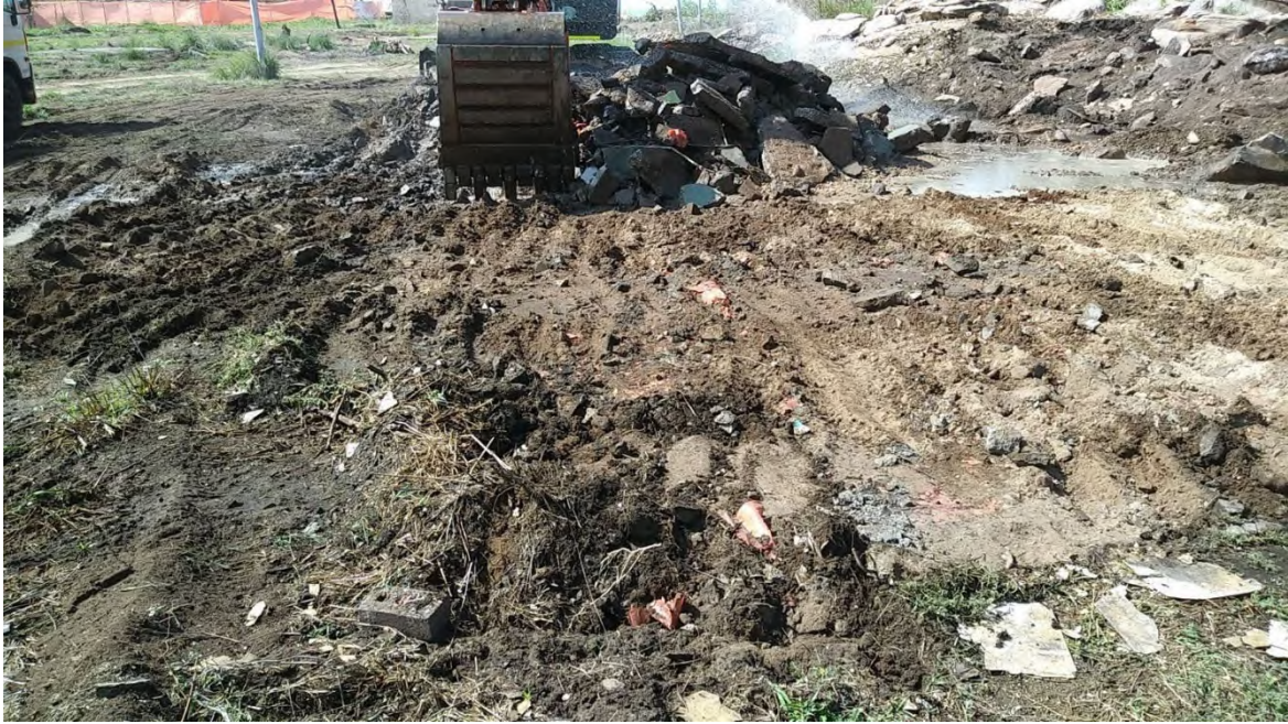
Asbestos contaminated soil removal from the rock wall (13/11/2018)
