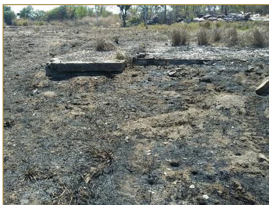
Photograph 15 – ACM debris on concrete pads across the site, with surrounding vegetation cover burnt, exposing further debris (July 2018)
