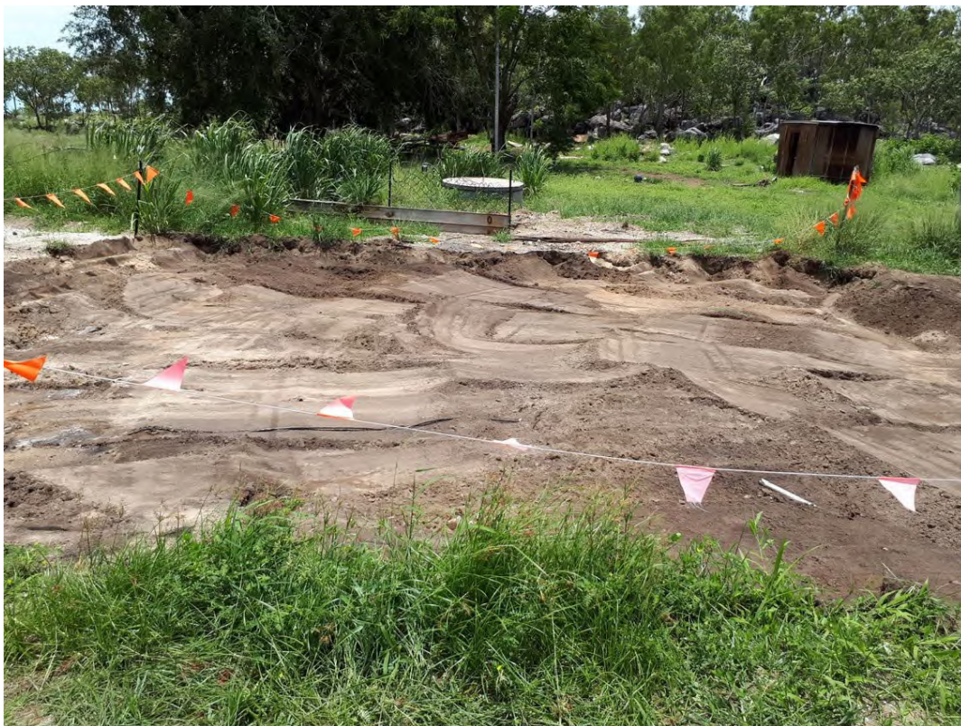
Additional soil removal area from soil exceedance location (Sample 190) (5/02/2019)
