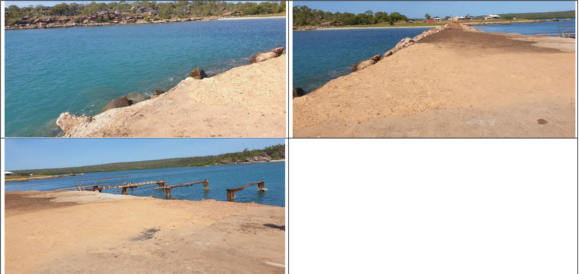
Photo 20 View from far end of Jetty looking south
