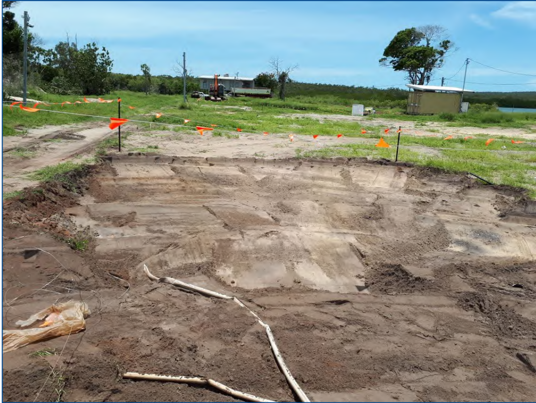
Additional soil removal area from soil exceedance location (Sample 160) (5/02/2019)
