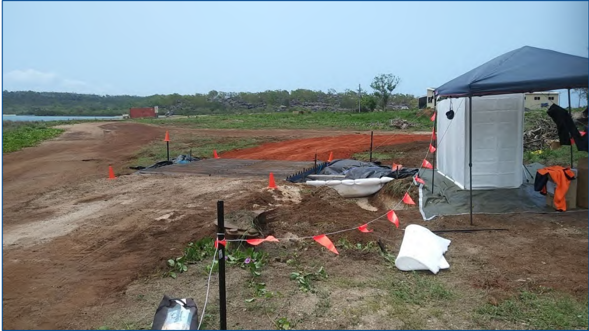
Rumble grid and wash water containment system construction, and decontamination unit – Homestead site (11/11/2018)
