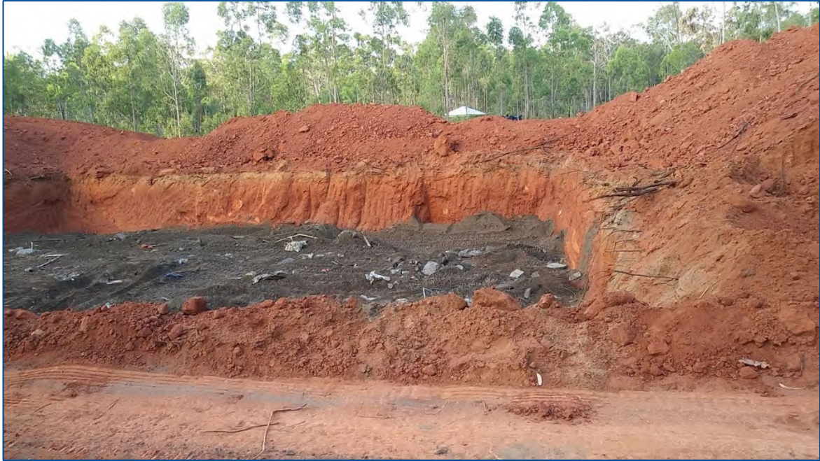
Disposal of asbestos waste within the containment cell (18/11/2018)
