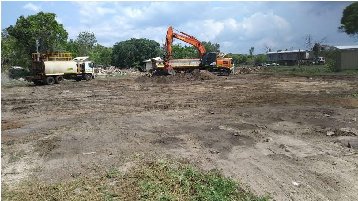
Asbestos contaminated soil removal from central site area, encompassing multiple redundant concrete foundations (19/11/2018)
