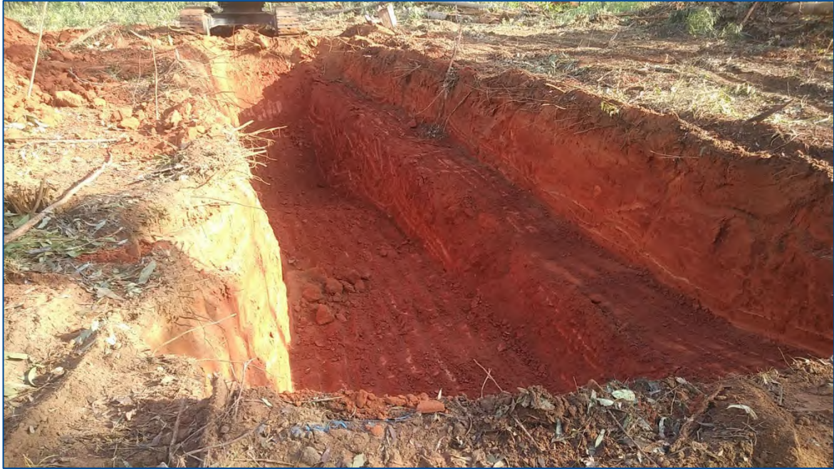
Containment cell construction (10/11/2018)
