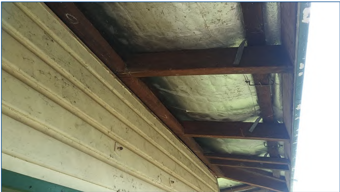
Removal of external eave linings of the Duplex Dormitory (12/11/2018)
