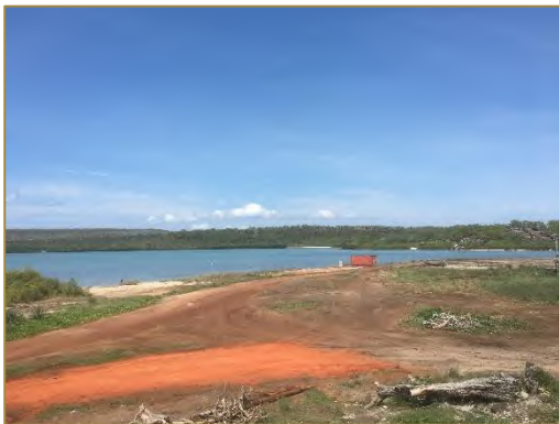
Photograph 5 – Bartalumba Bay Homestead post asbestos removal works
