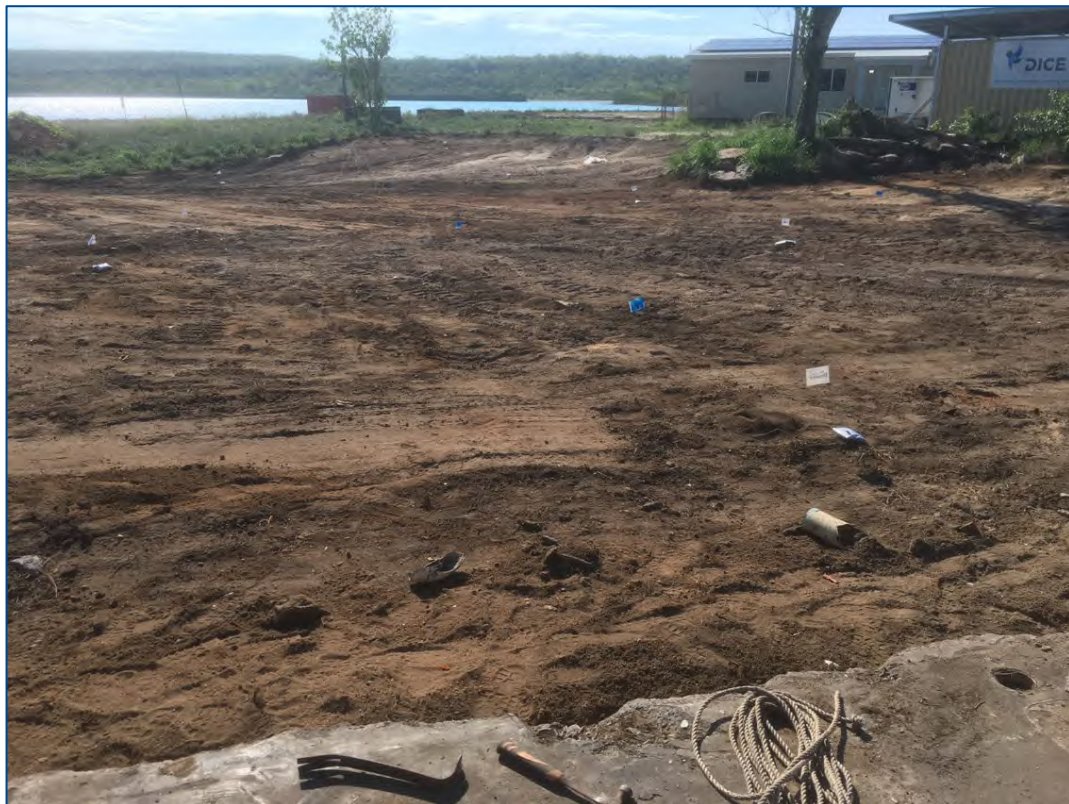
Final site condition looking north-west across central site area (22/11/2018)
