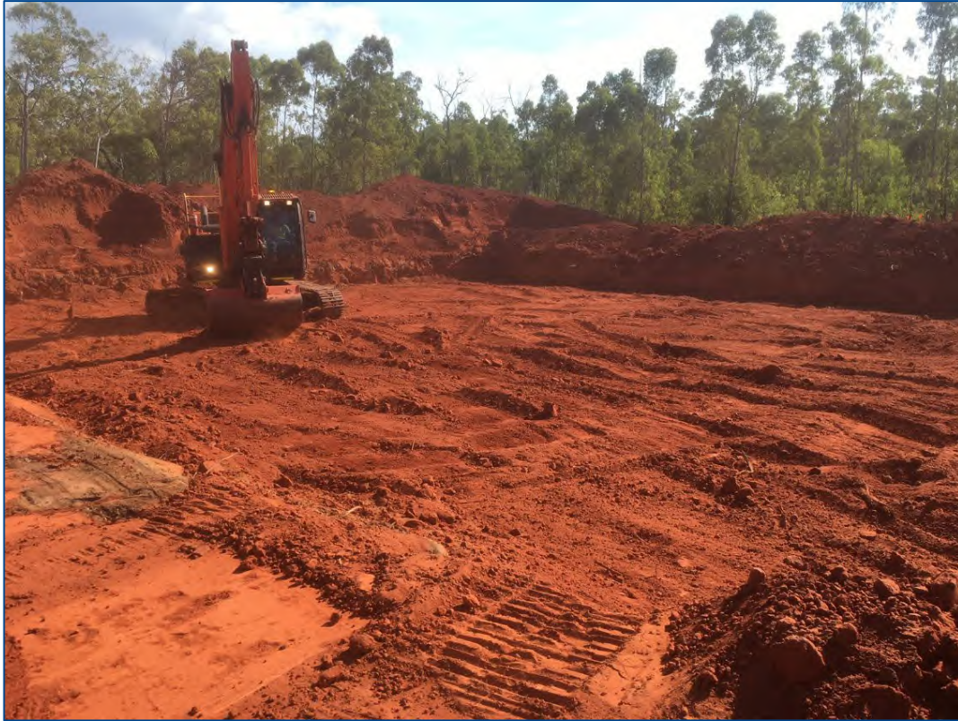
Progressive cap compaction (23/11/2018)
