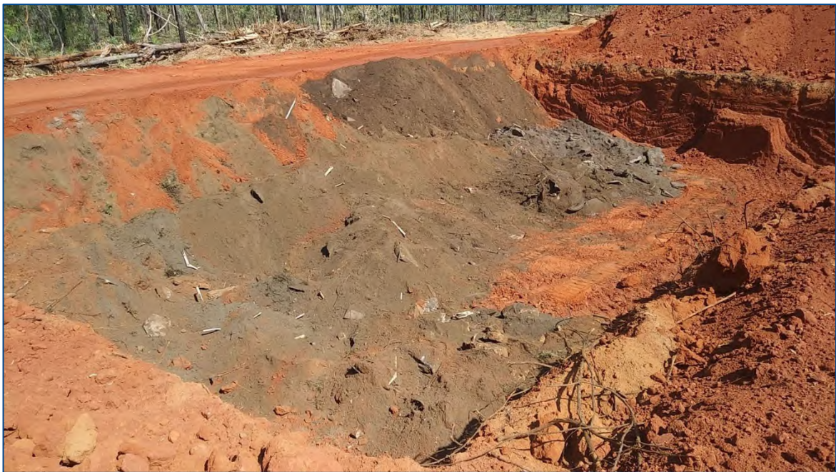
Disposal of asbestos waste within the containment cell (16/11/2018)
