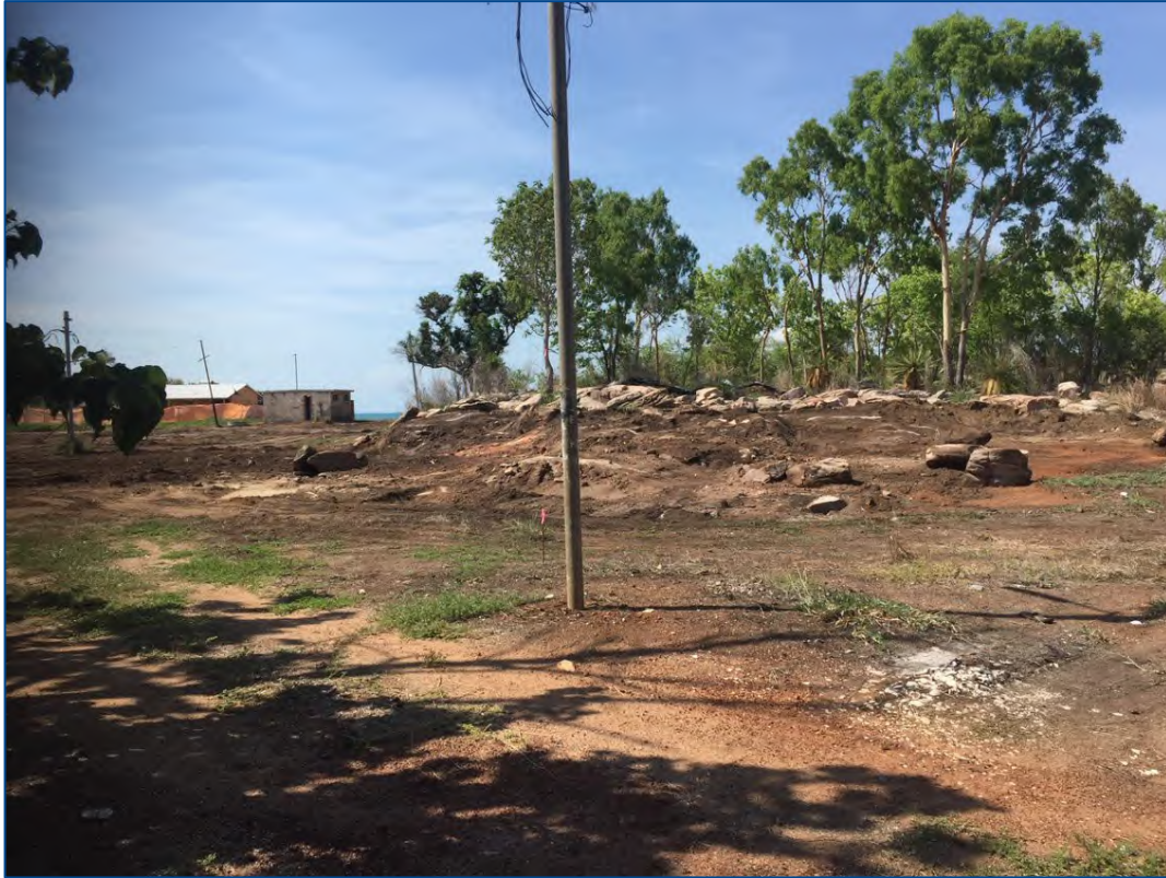
Asbestos contaminated soil removal from rock wall area (20/11/2018)
