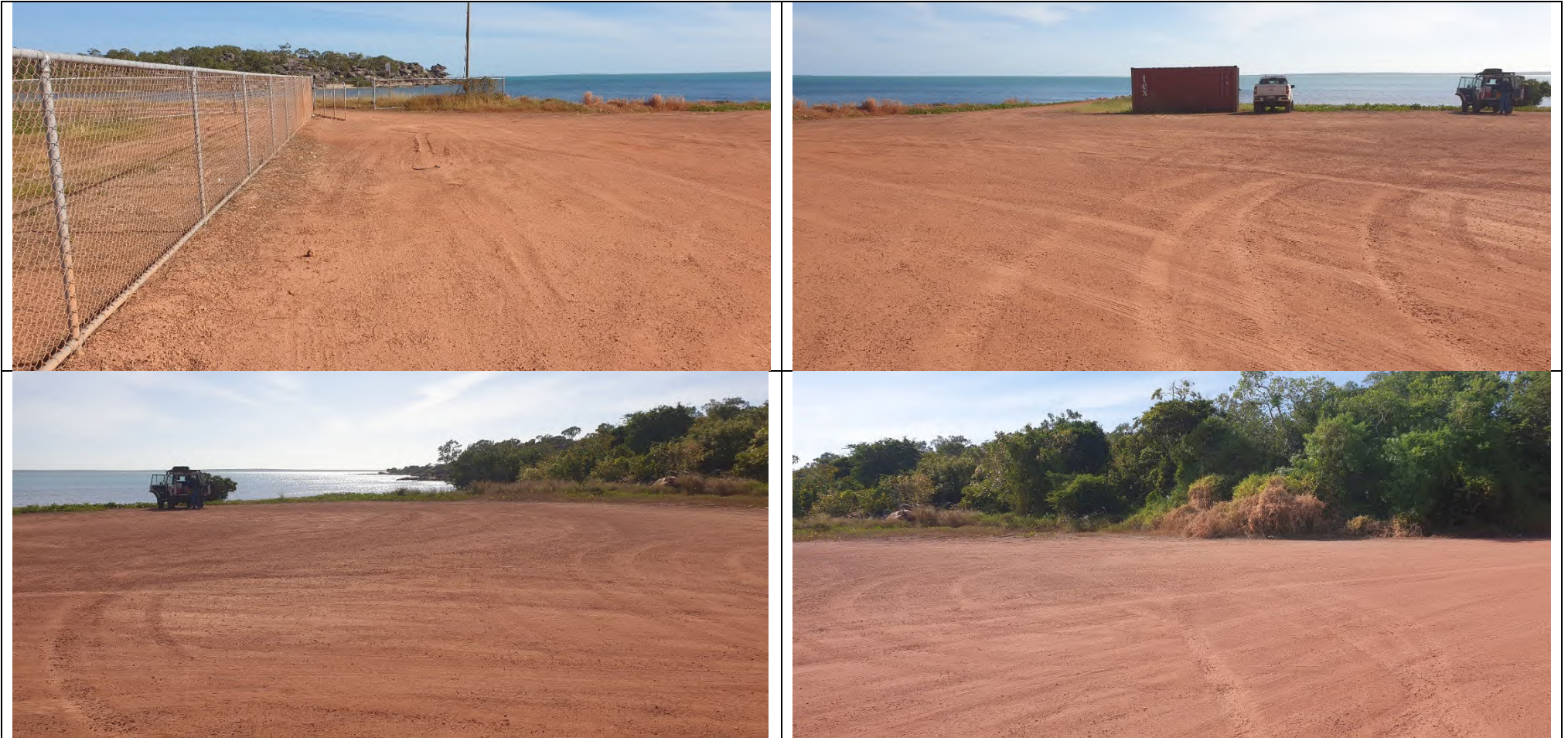
Photo 14 Former Recreation Club area looking north
