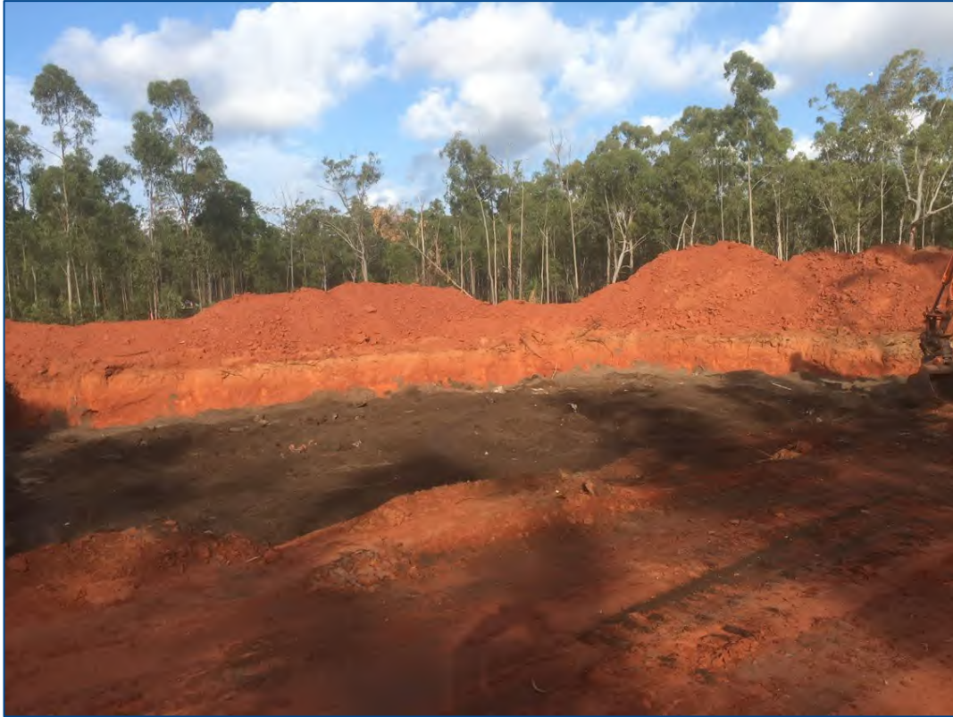
Containment cell prior to capping (23/11/2018)
