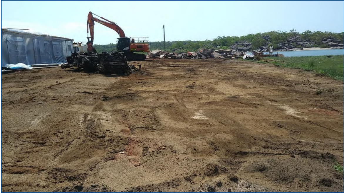
Asbestos contaminated soil removal from north of the Recreation Club (17/11/2018)
