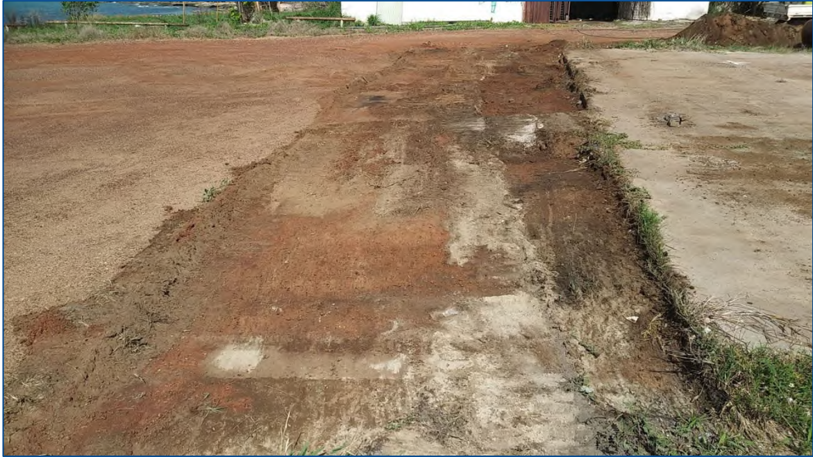
Completed removal around redundant concrete foundation No. 4 (12/11/2018)
