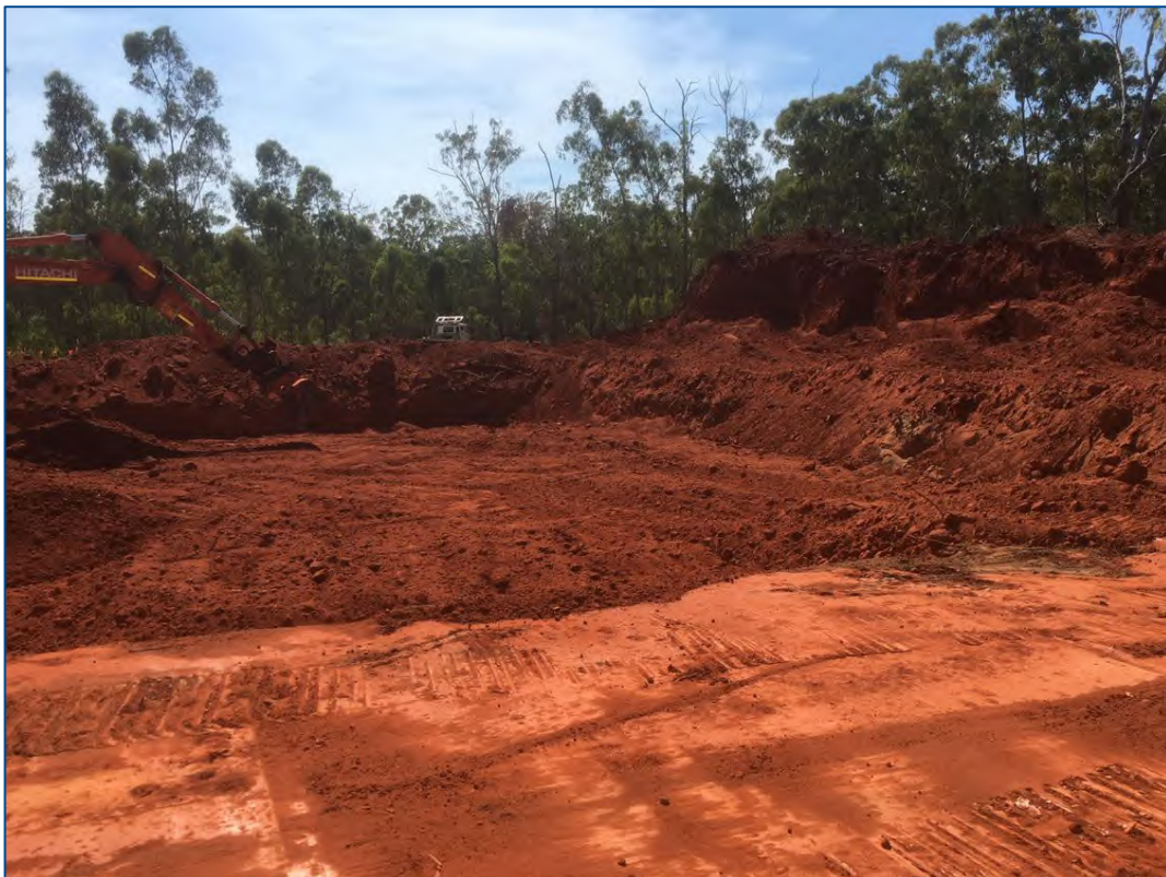
Capping in progress (23/11/2018)
