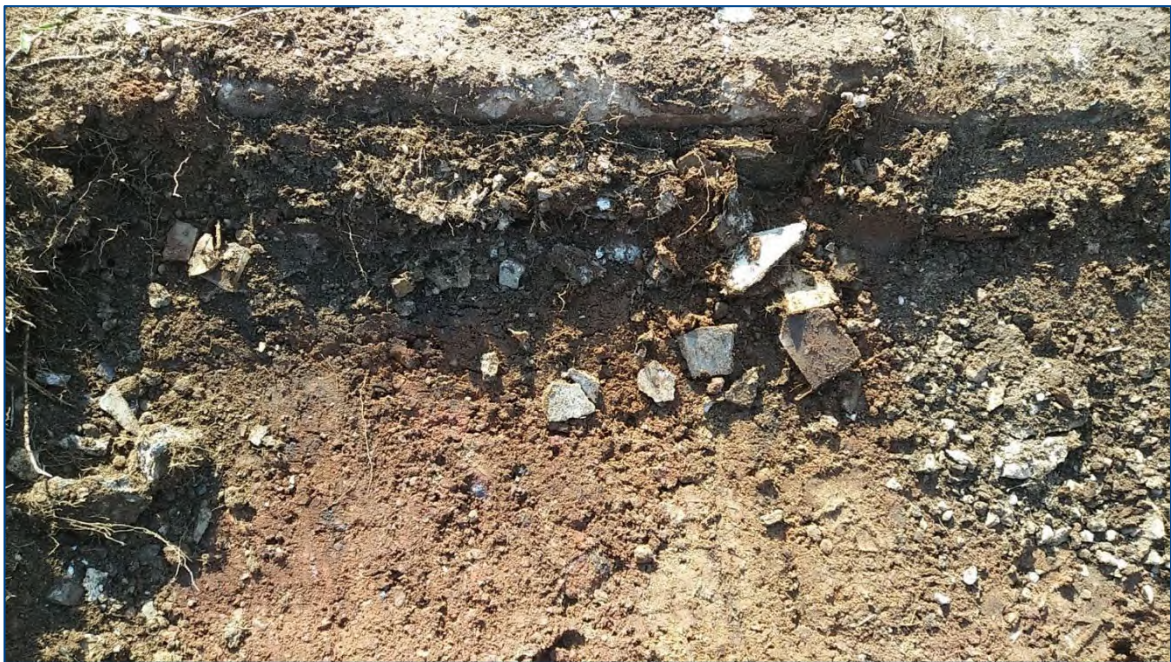
Asbestos contaminated soil removal around redundant concrete foundation No. 4 (12/11/2018)
