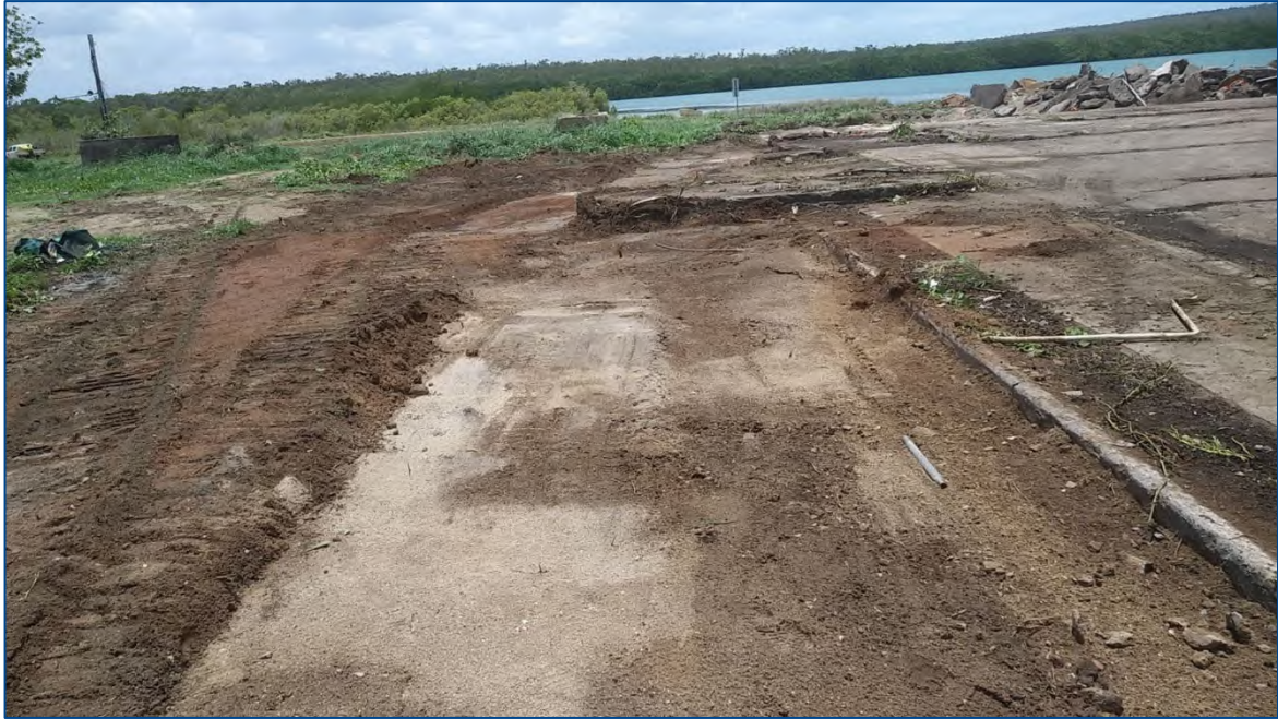
Asbestos contaminated soil removal from around the Redundant Concrete Foundation No.1 (16/11/2018)
