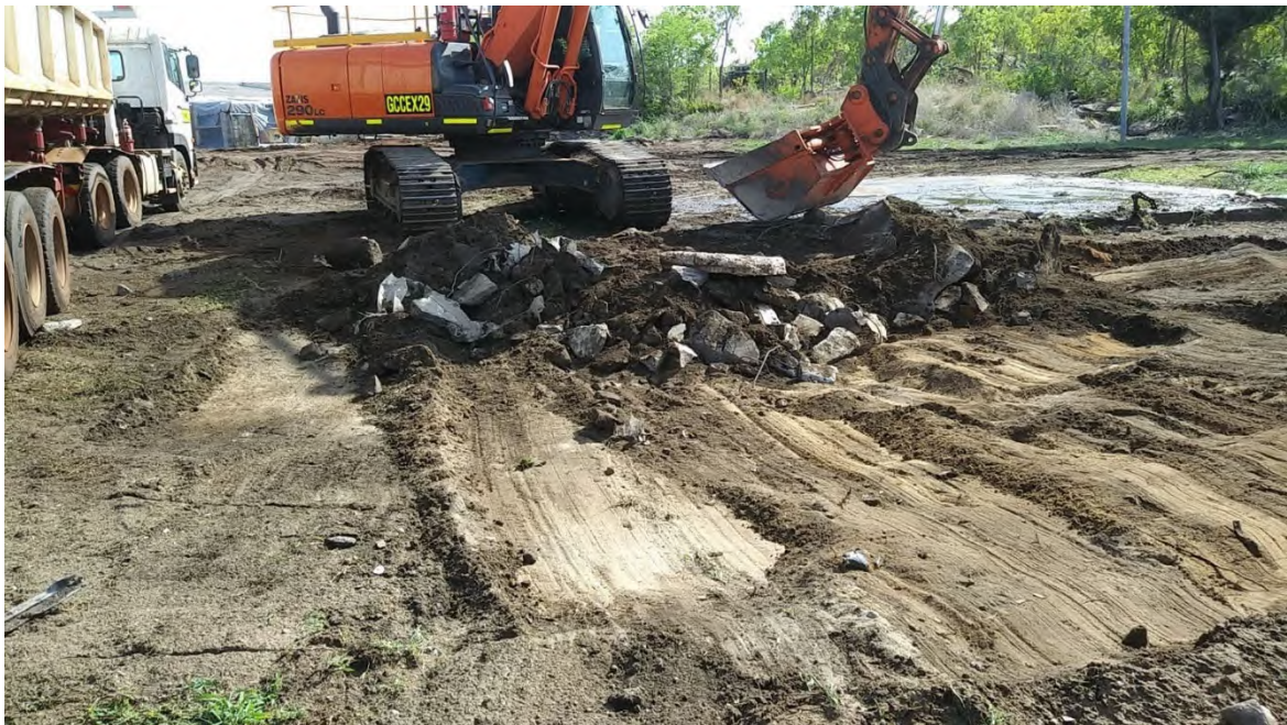
Asbestos contaminated soil removal from redundant concrete foundation No. 5 (18/11/2018)
