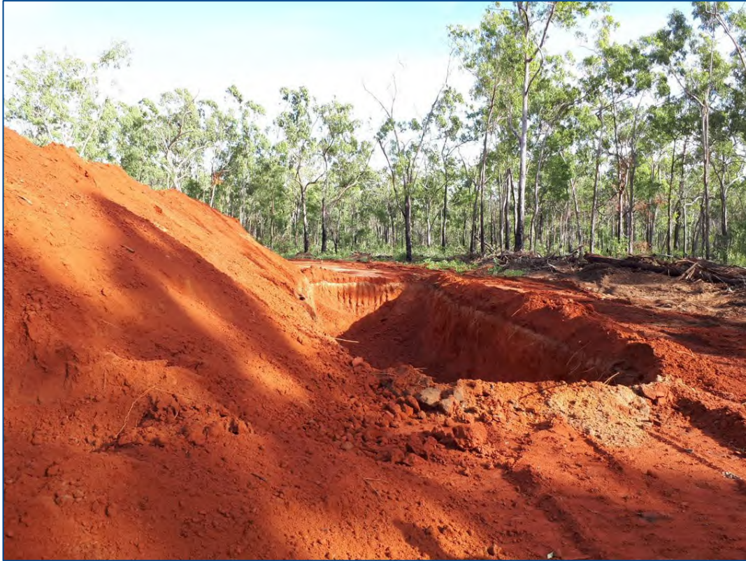
Expansion of containment cell (4/02/2019)
