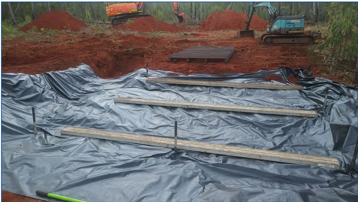
Rumble grid and wash water containment system construction – Containment Cell site (10/11/2018)
