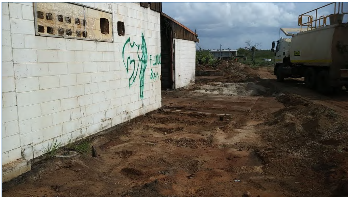
Asbestos contaminated soil removal from around the Recreation Club (13/11/2018)
