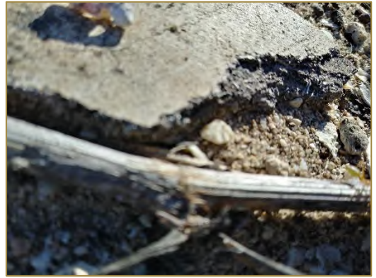
Photograph 14 – ACM debris on concrete pads across the site
