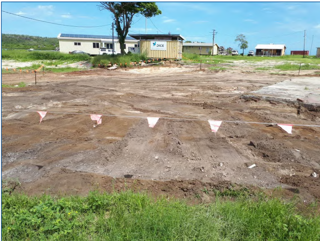
Additional soil removal area from soil exceedance locations (Samples 177, 178, 179, 180, 181, 183) (6/02/2019)
