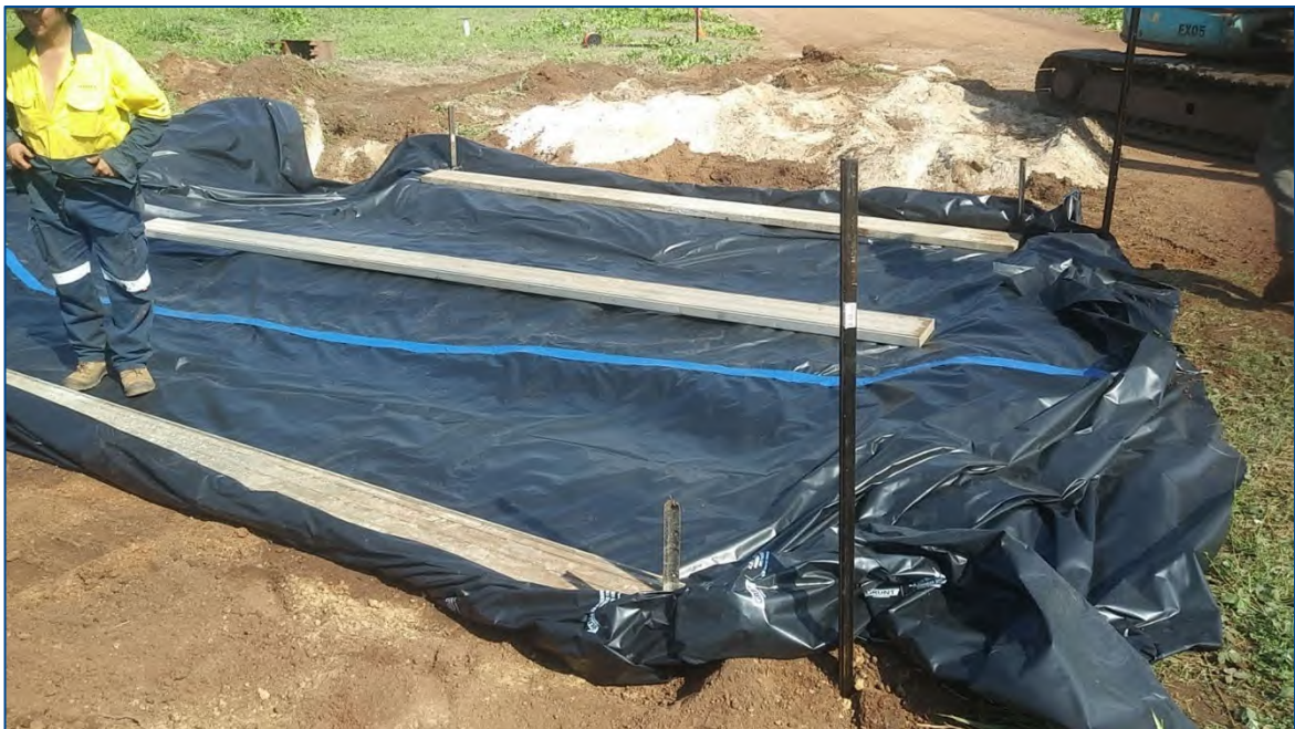
Rumble grid and wash water containment system construction – Homestead site (10/11/2018)
