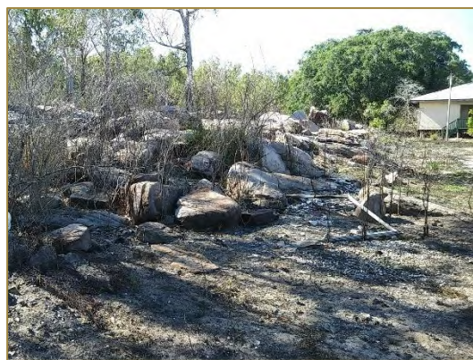
Photograph 21 – ACM debris spread across area encompassing the rock wall, north of the Duplex Dormitory
