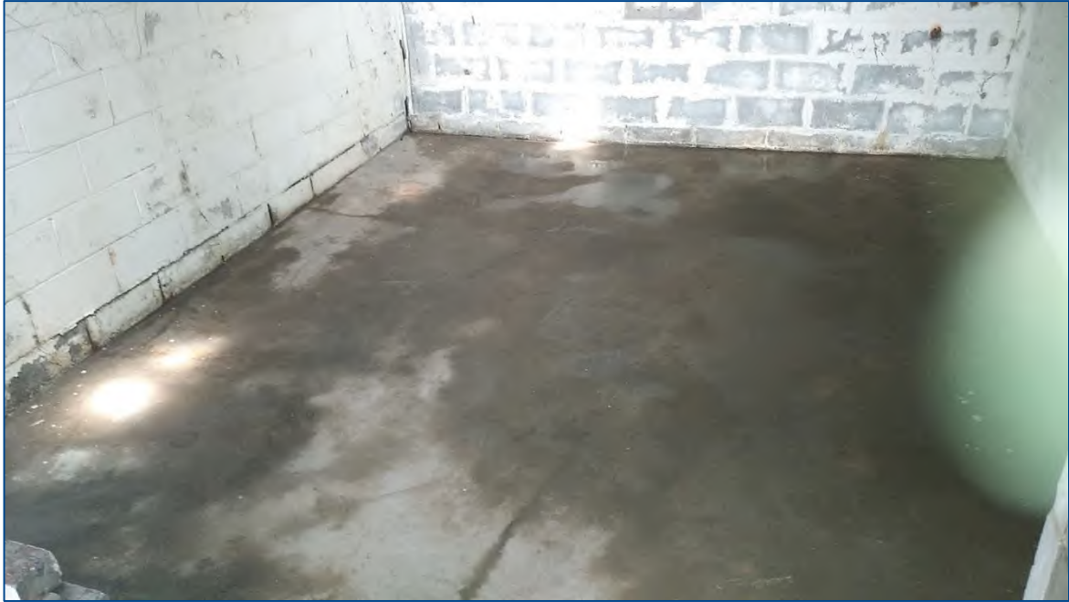
Decontaminated room of Recreation Club (18/11/2018)
