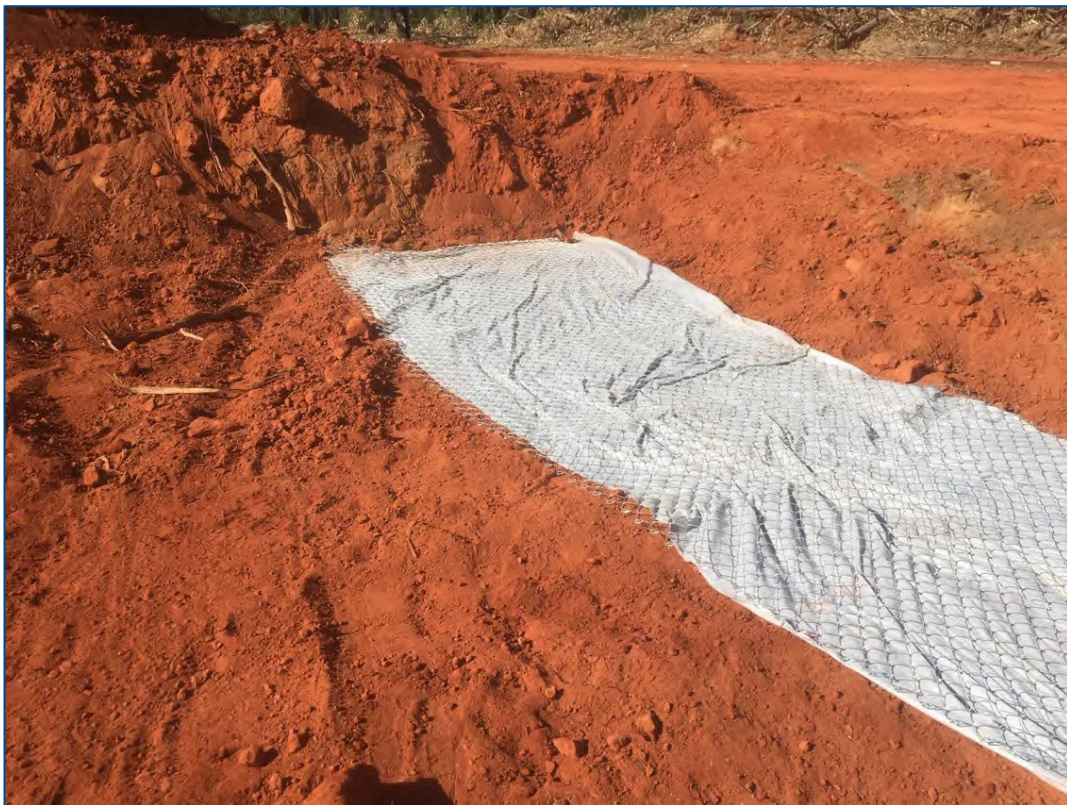
Geofabric and high visibility mesh fencing material over contaminated material (23/11/2018)
