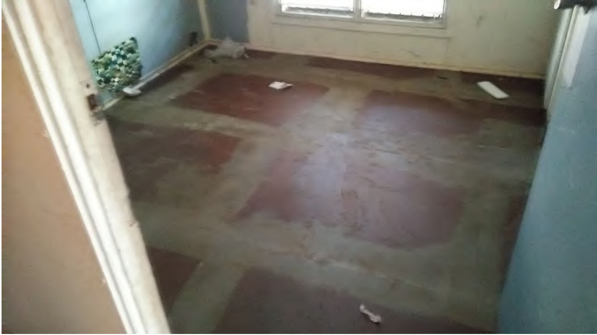
Completed of internal vinyl tile from Duplex Dormitory (12/11/2018)
