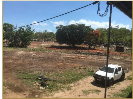
Photograph 2 – Bartalumba Bay Homestead post asbestos removal works
