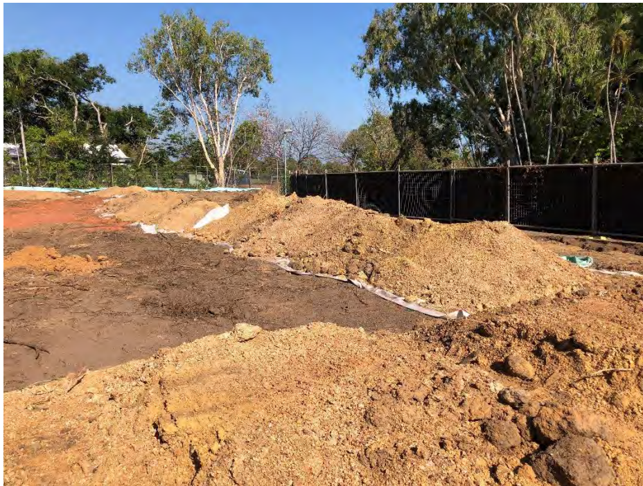
Plate 5: Processed "clean" stockpiles generated during trenching activities, stored on geofabric.
