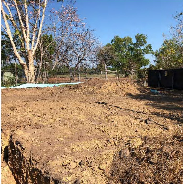
Plate 4: Proposed outdoor play area (south-west corner of the site). Additional, shallow trenching on a grid basis to confirm absence of ACM completed in this area following identification and removal of additional corrugated sheet fencing
