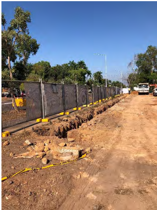
Plate 2: Trenching to remove corrugated asbestos fencing, southern site boundary.
