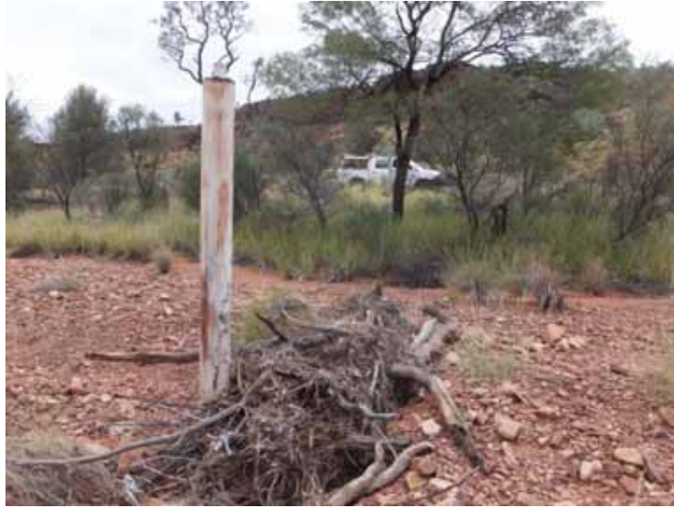
PHOTOGRAPH 6: VIEW OF BORE RN16354 LOCATED IN THE CREEK BED. IT WOULD BE PREFERABLE TO CLEAR A SITE ON THE BANK NEAR THE VEHICLE AND DRILL A NEW BORE TO 120M DEPTH.
