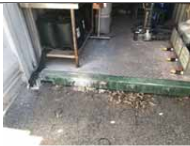
Photo: Evidence of effluent overflow onto ground from door of control/dosing room.
