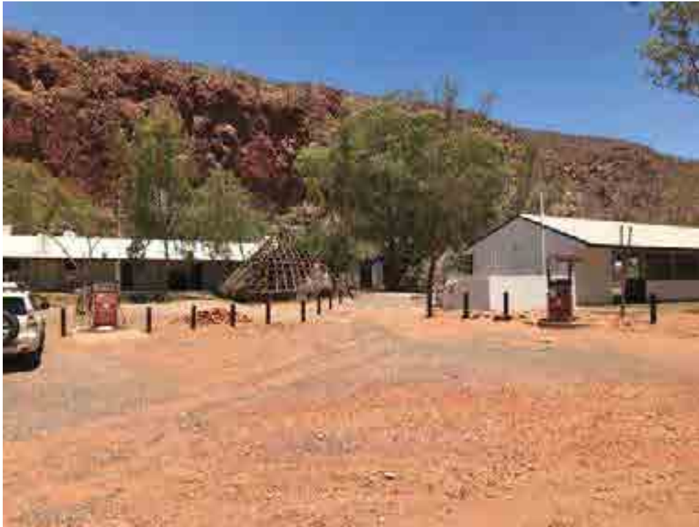
Fuel systems at edge of carpark prior to removal
