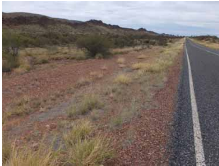
PHOTOGRAPH 4: NAMATJIRA DRIVE CH. 94. TYPICAL VIEW OF TABLE DRAIN AND VERGE. CONSTRUCTING A PIPE LINE ALONG THE ROAD WOULD REQUIRE TRENCHING IN VERY ROCKY SOIL. IMPORTED BEDDING AND PIPE EMBEDMENT MATERIAL WILL BE REQUIRED.
