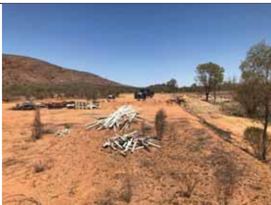
Photo: Scrap metal stockpiled on the site.
