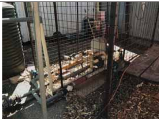
Photo: Old wastewater treatment system. Also several tanks.
