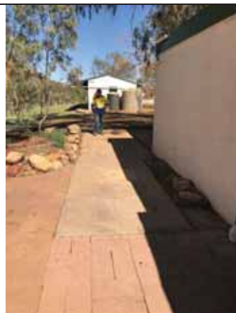
Photo: Concrete filled lid openings, possible old septic tank.
