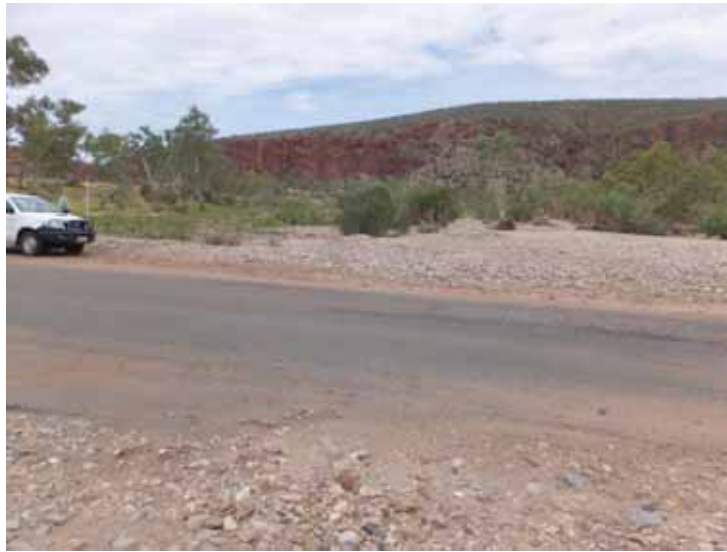
PHOTOGRAPH 2: NAMATJIRA DRIVE CHAINAGE (CH.) 85.7. VIEW OF THE FINKE RIVER CROSSING. THIS RIVER PROVIDES A SUBSTANTIAL OBSTACLE FOR THE CONSTRUCTION OF A PIPE LINE UNDER THE RIVER BED. ANY WORK WOULD REQUIRE AN AAPA AUTHORITY CERTIFICATE BECAUSE OF KNOWN SACRED SITES NEARBY.
