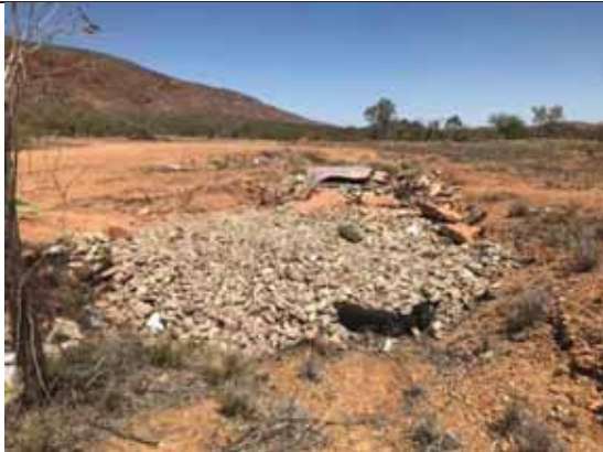
Photo: Current part of trench in foreground and previously filled/covered small area behind. This is mostly tiles and concrete rubble.
