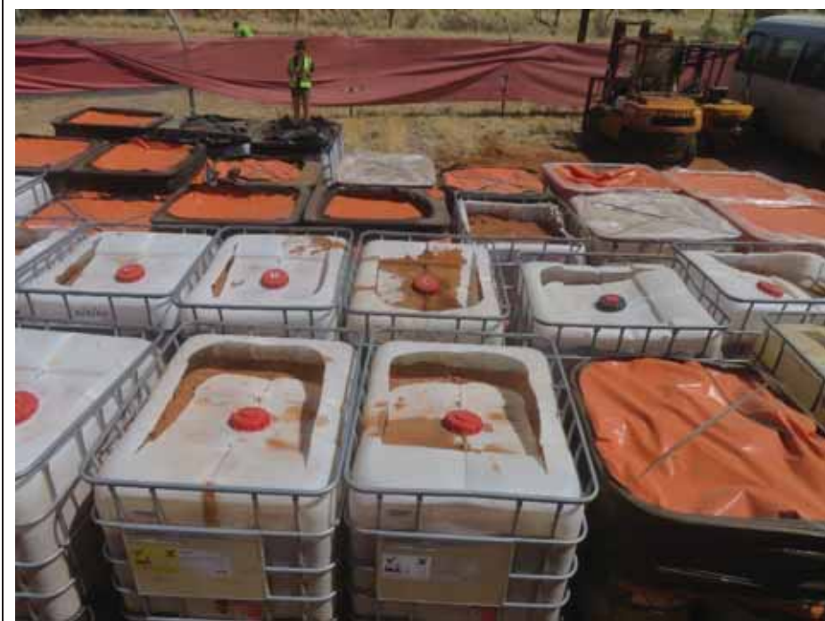
Image 14. Contaminated excavated soil in storage pods and IBCs prior to disposal.
