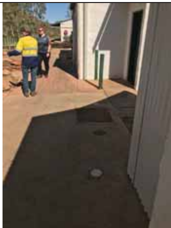
Photo: Grease trap cover.
