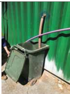
Photo: Evidence of effluent overflow onto ground from door of control/dosing room.
