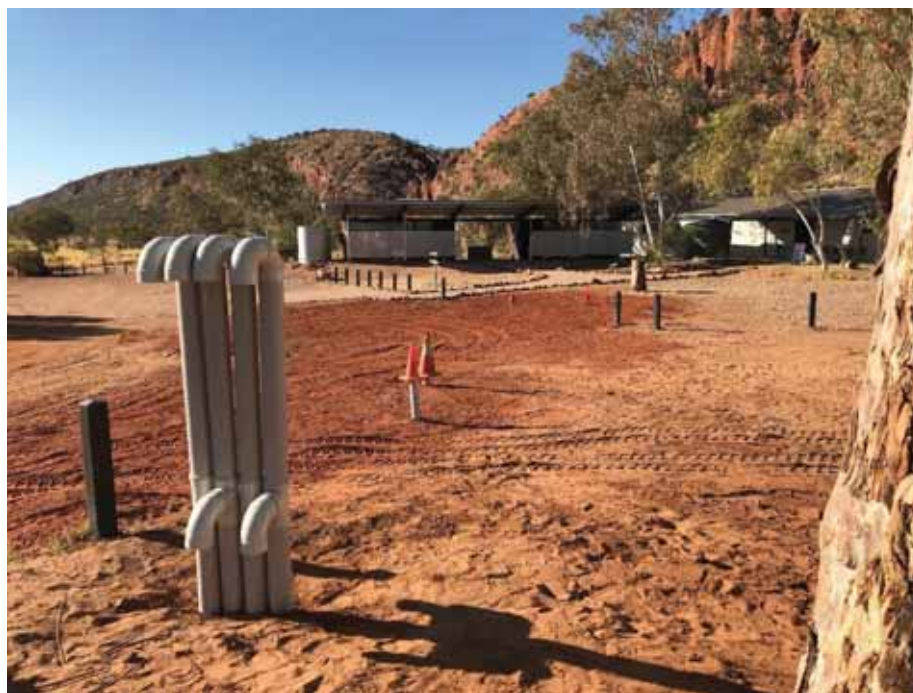
Image 12. Opal petrol pit location after it had been backfilled with clean imported soil with visibly exposed vent pipes.
