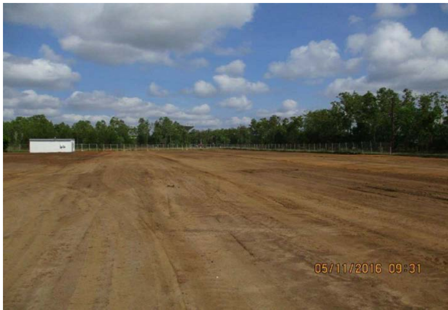
Photo 8: Finished surface after re-compaction
