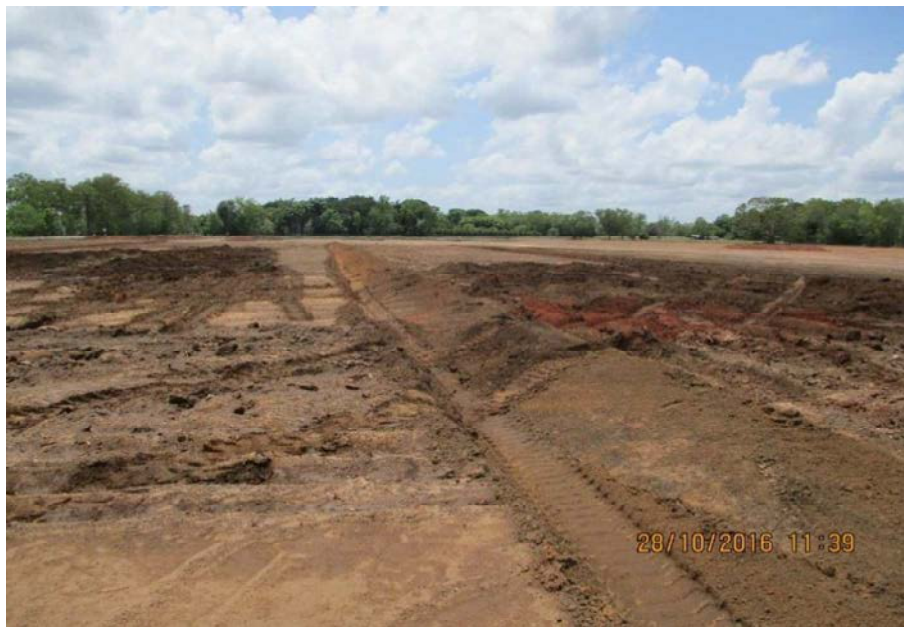
Photo 6: Forming a drain to the east end of the site during mixing to allow rainfall to runoff more effectively
