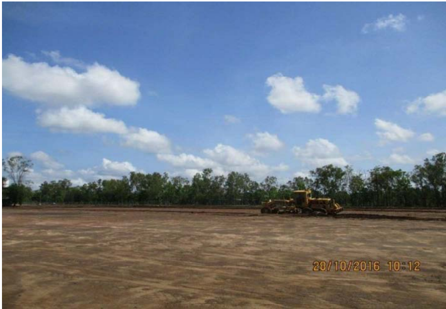
Photo 4: Tying on the MD site
