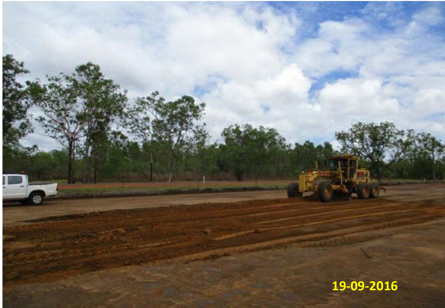
Photo 3: Trial mixing area
