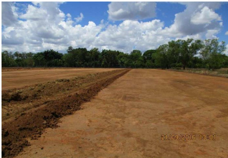
Photo 4: Topsoil, stripped and winrowed prior to removal from the SD zone
