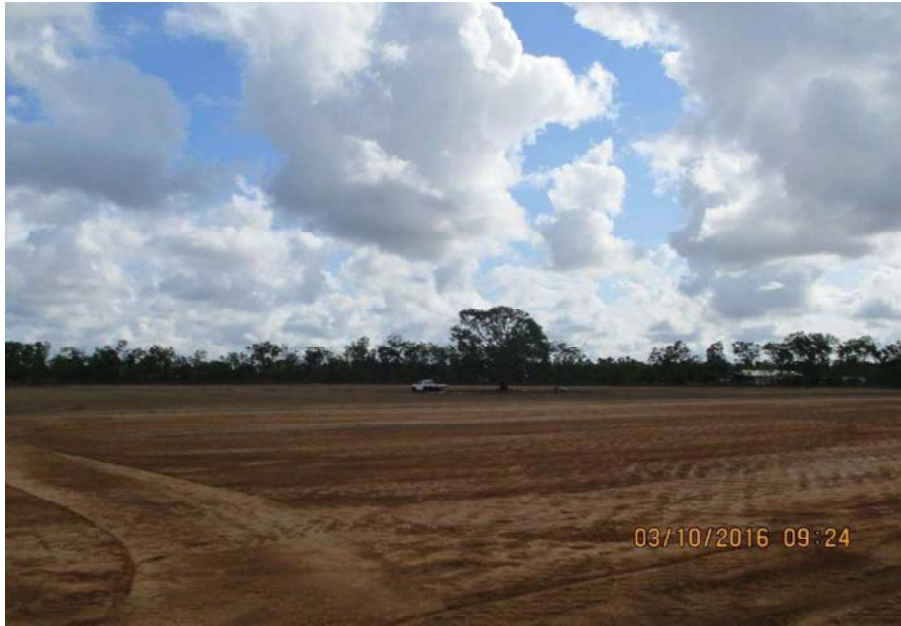
Photo 7: Overview of SD Zone after re-compaction and sealed, post mixing
