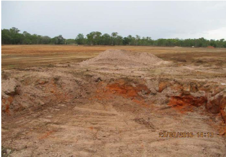
Photo 7: Partially backfilled hotspot excavation
