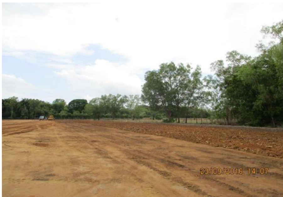
Photo 6: Tyned area prior to mixing (RHS)
