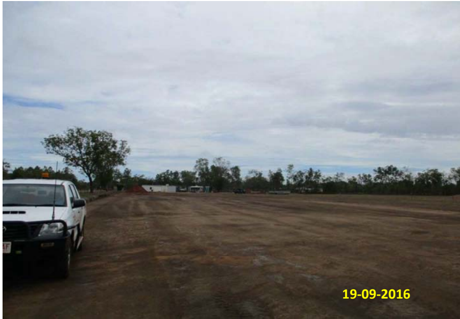
Photo 1: Typical site surface post topsoil stripping
