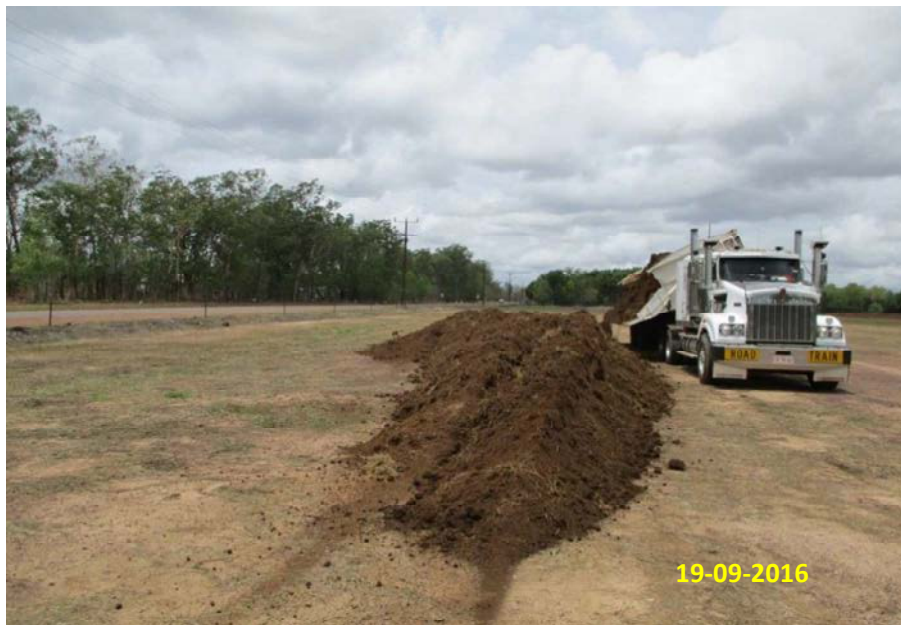
Photo 2: Topsoil stockpile on the MD site
