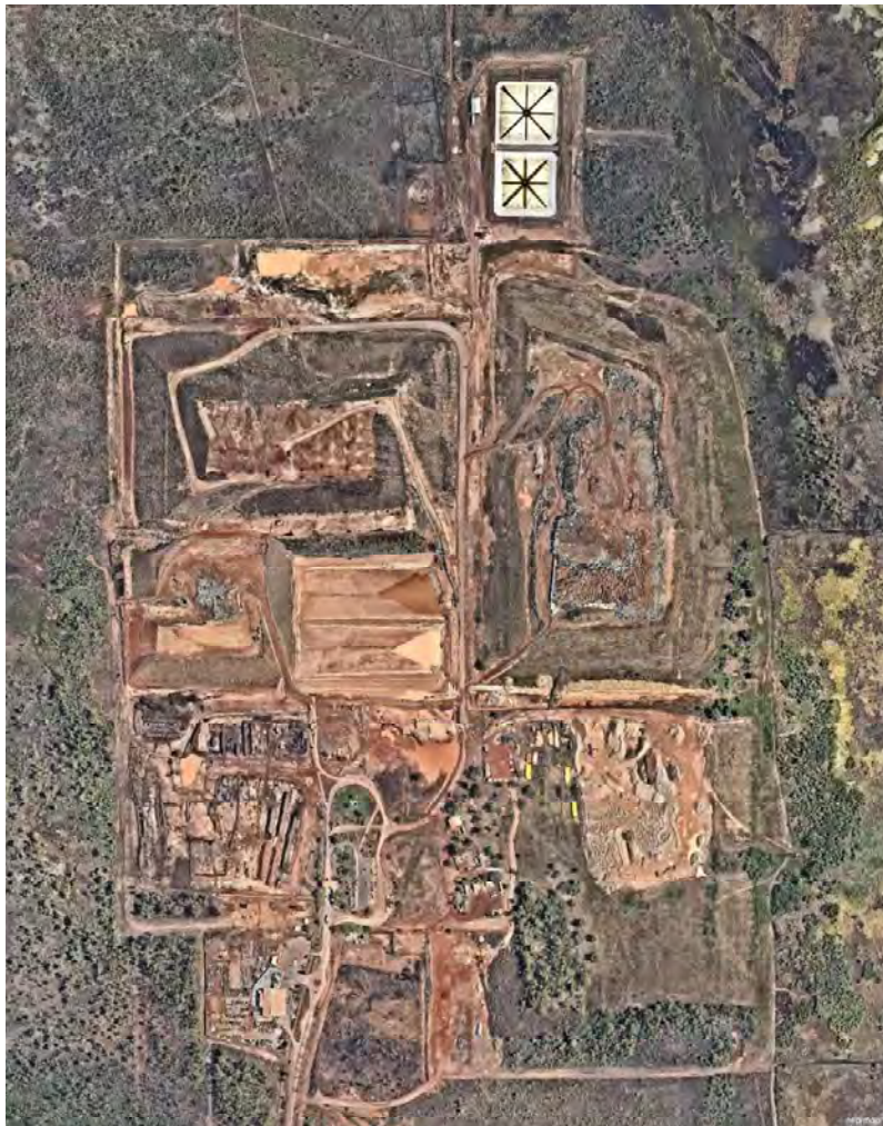
Figure 1-1 Shoal Bay Waste Management Facility
