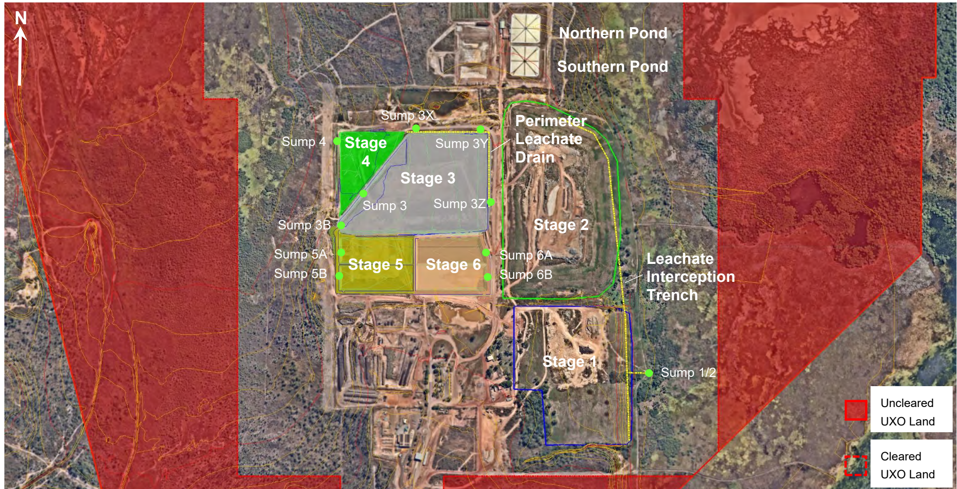
Figure 3: Constructed Landfill Waste Cells and Leachate Collection Systems
