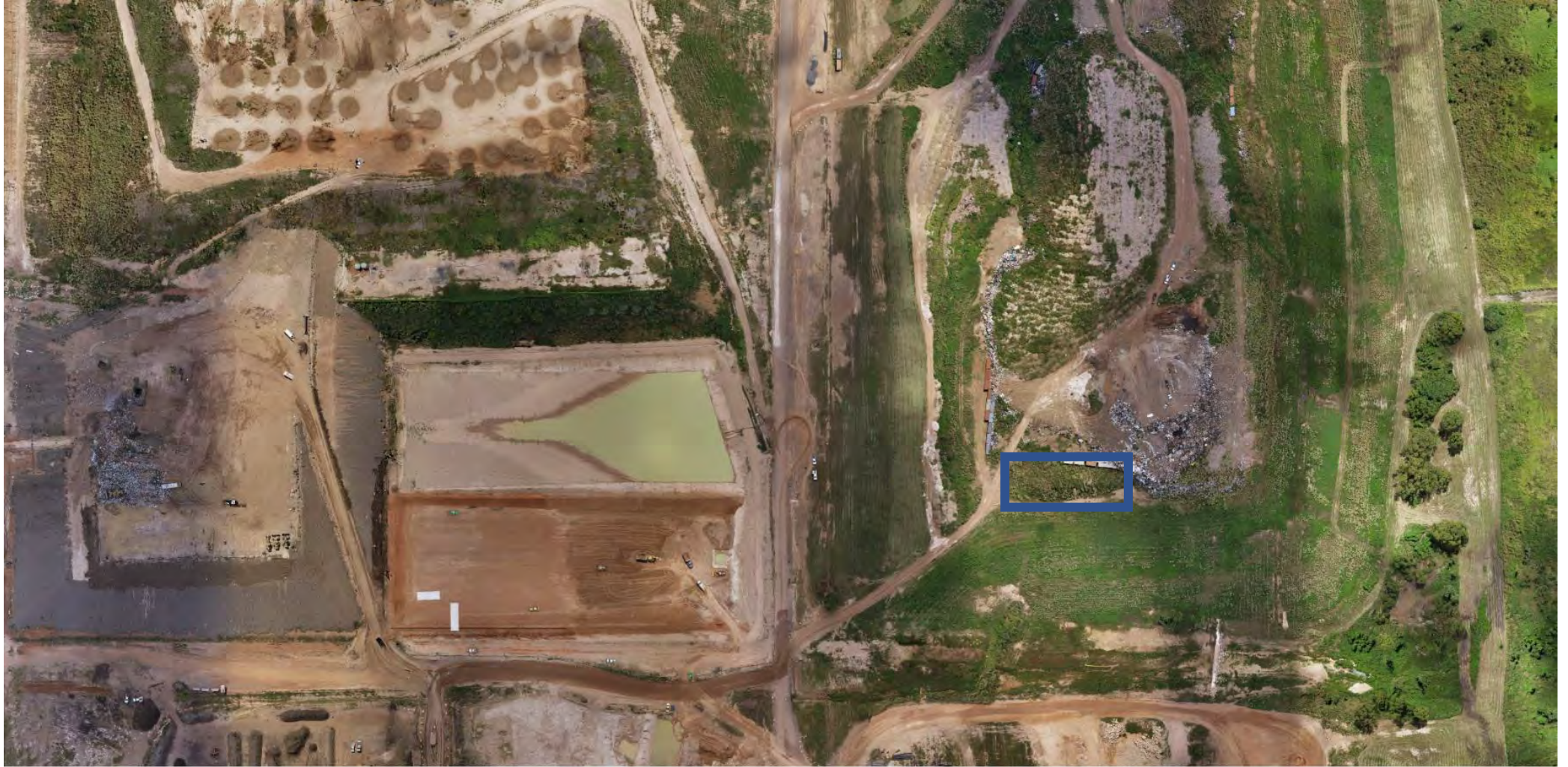
Figure 1. Shoal Bay Waste Management Facility
