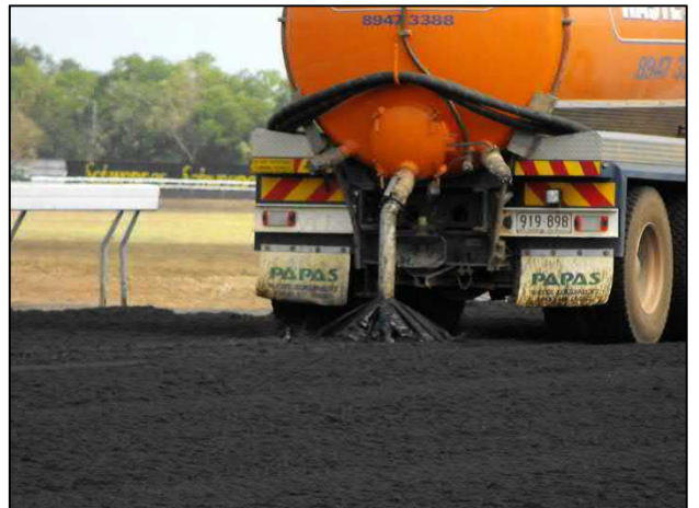
Photo 7: Application of oil to track surface.
