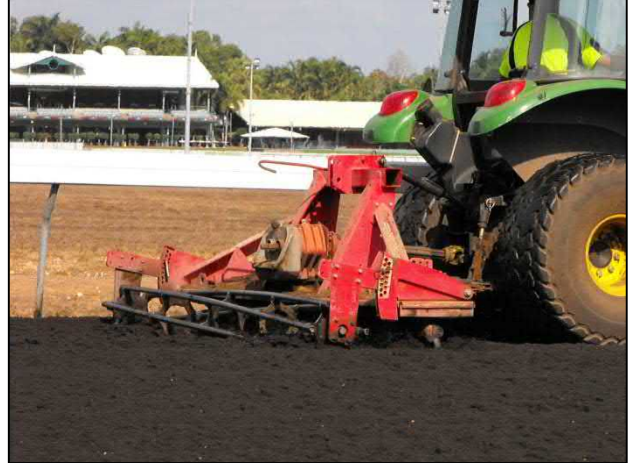
Photo 5: Tilling of track surface.
