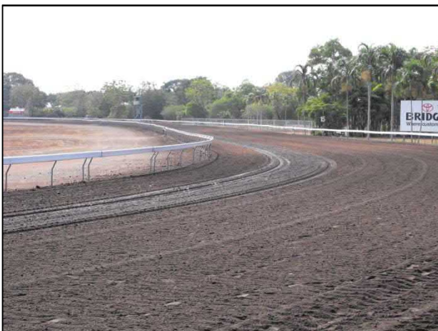
Photo 8: Inner track marks indicate latest application and tilling of track.
