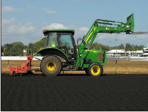
Photo 4: Tilling of track surface during oil application.
