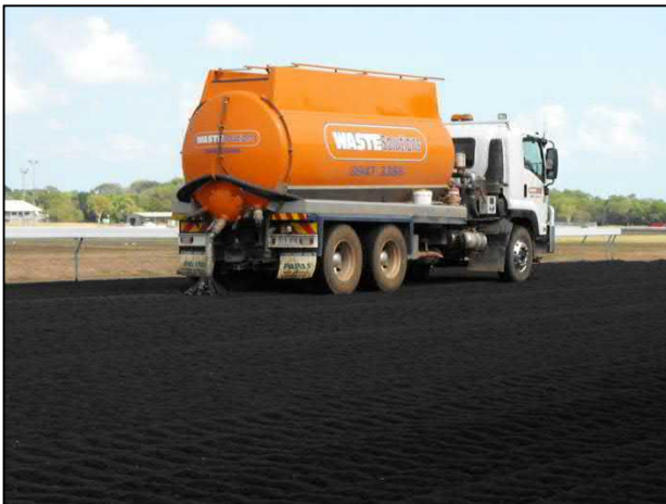
Photo 6: Application of oil to the track surface.
