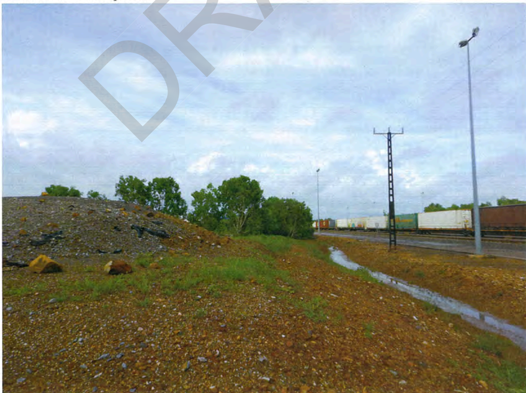
Photograph 2: Stockpiled material facing west. Earthen stormwater drain visible on far right of image, flowing west.
