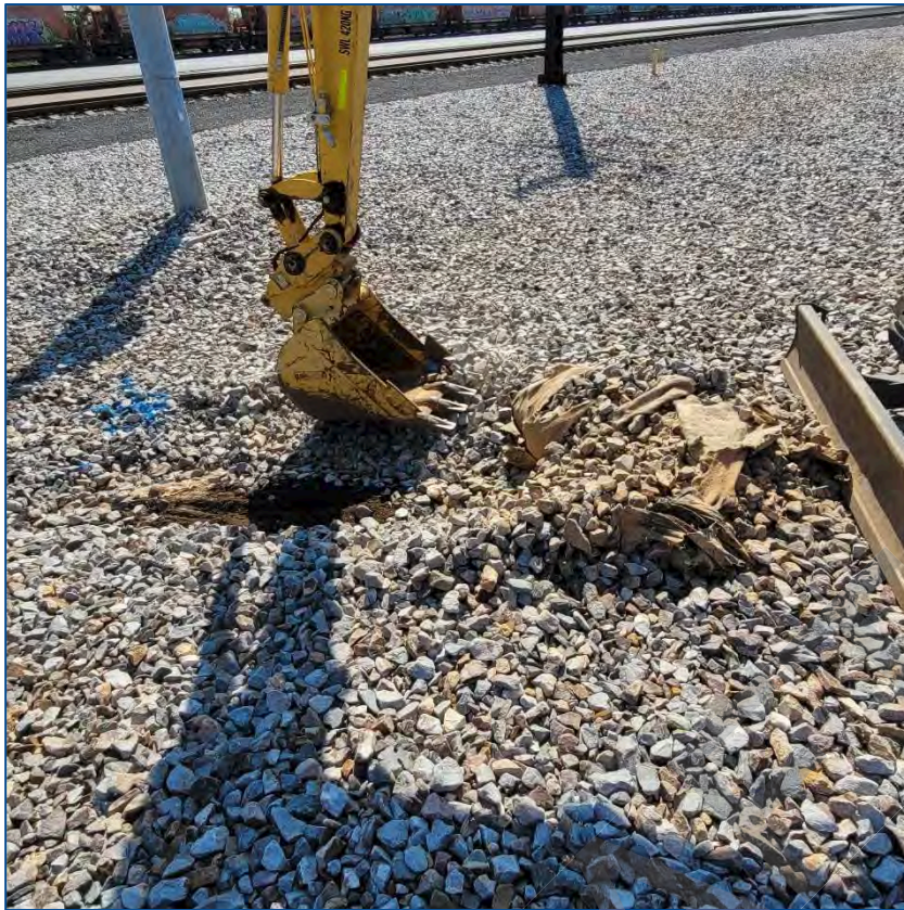
Photograph 3: View of rail ballast surface at A2_TP01 in Area 2
