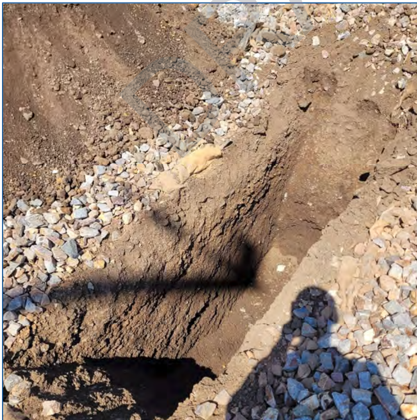
Photograph 4: View of A2_TP02 in Area 2
