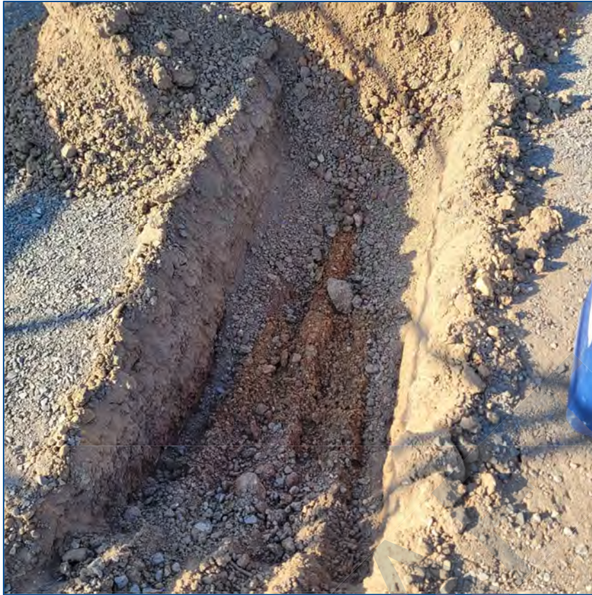
Photograph 6: View of A3_TP01 in Area 3
