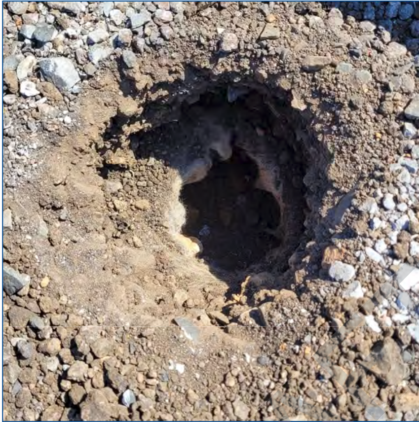
Photograph 1: View of borehole with ballast and geofabric material in Area 1
