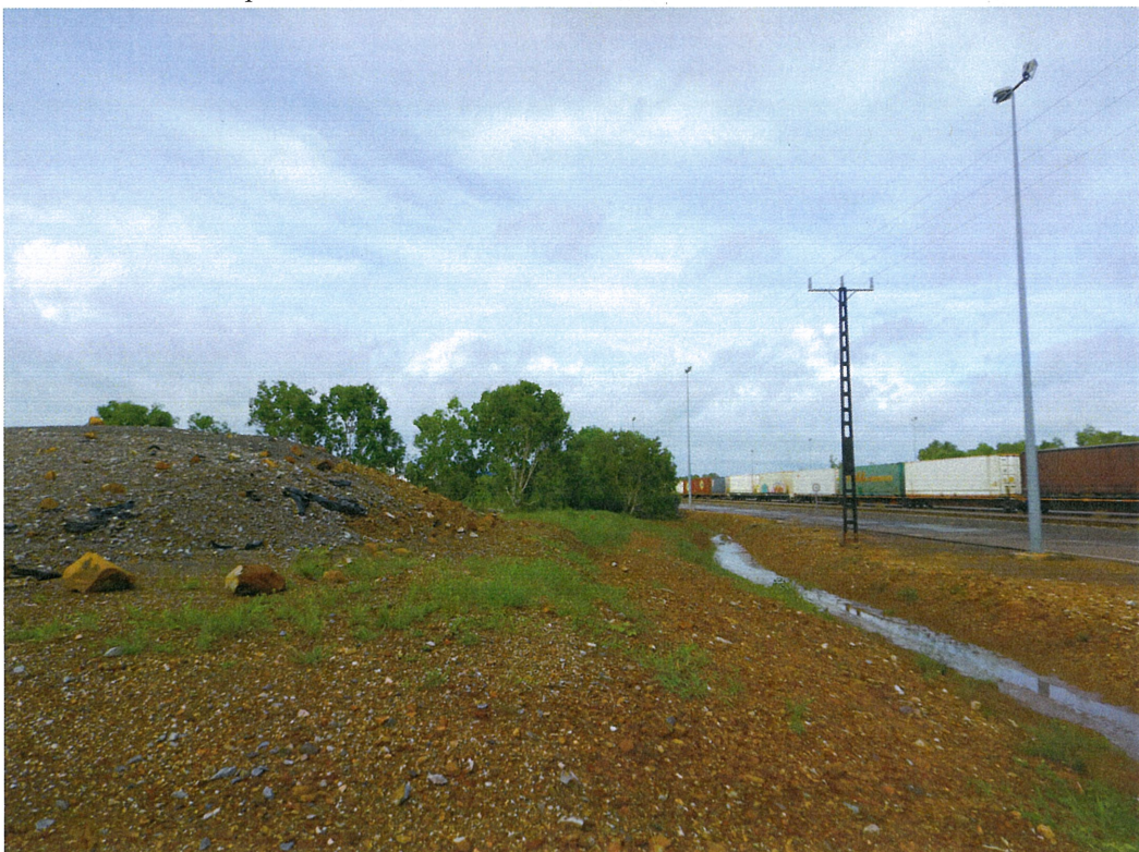
Photograph 2: Stockpiled material facing west. Earthen stormwater drain visible on far right of image, flowing west.
