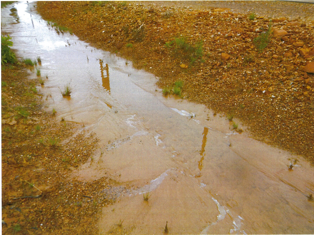
Photograph 5: Earthen stormwater drain located north of the stockpile. Visible hydrocarbon-like sheen visible in water and on surrounding ground surfaces.
