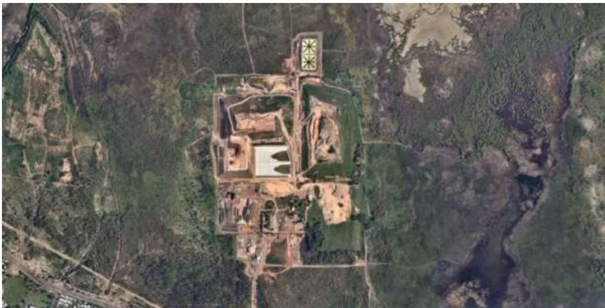
Figure 1: Shoal Bay Waste Management Facility (NearMaps 2020)
