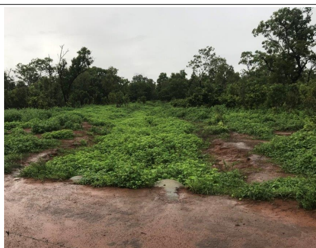
SW04 Discharge culvert (NW Boundary)
