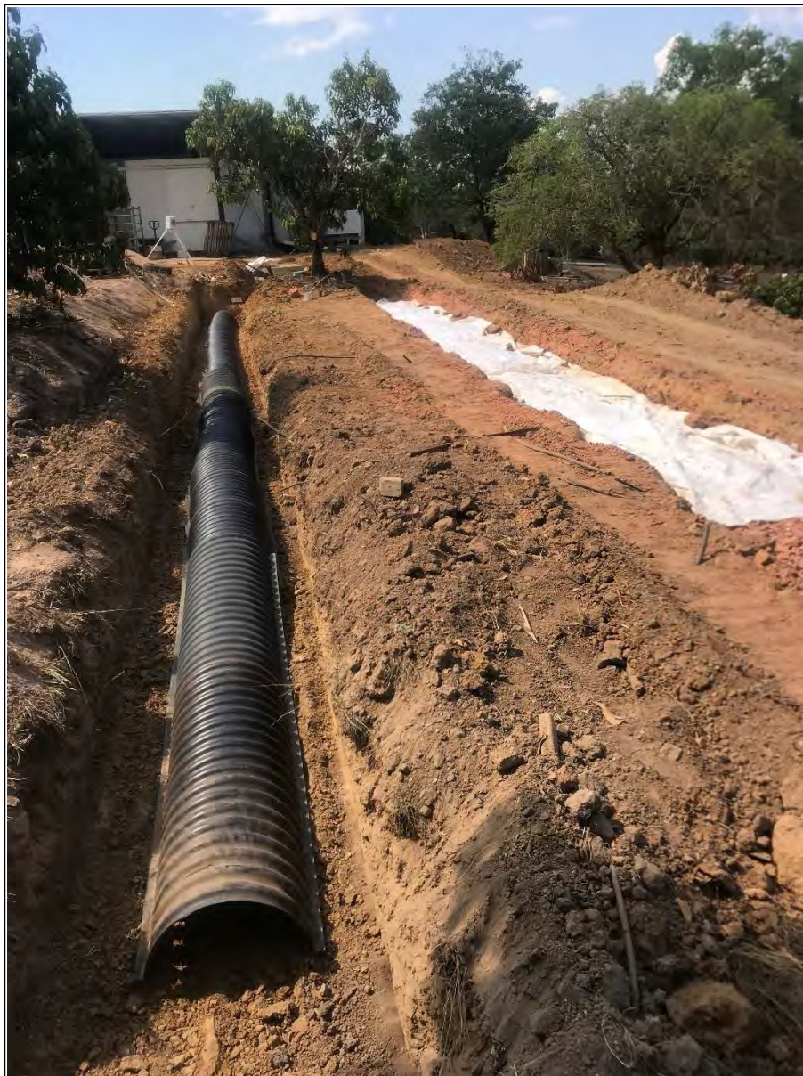
Image 7: Construction of soil absorption trenches
