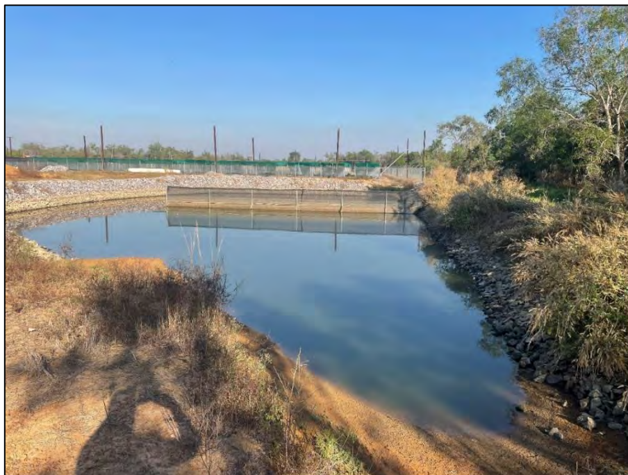
Image 5: Waste stabilisation pond showing discharge outlet in foreground
