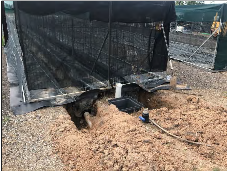
Image 4: Inlet works to improve water distribution into the finishing pens
