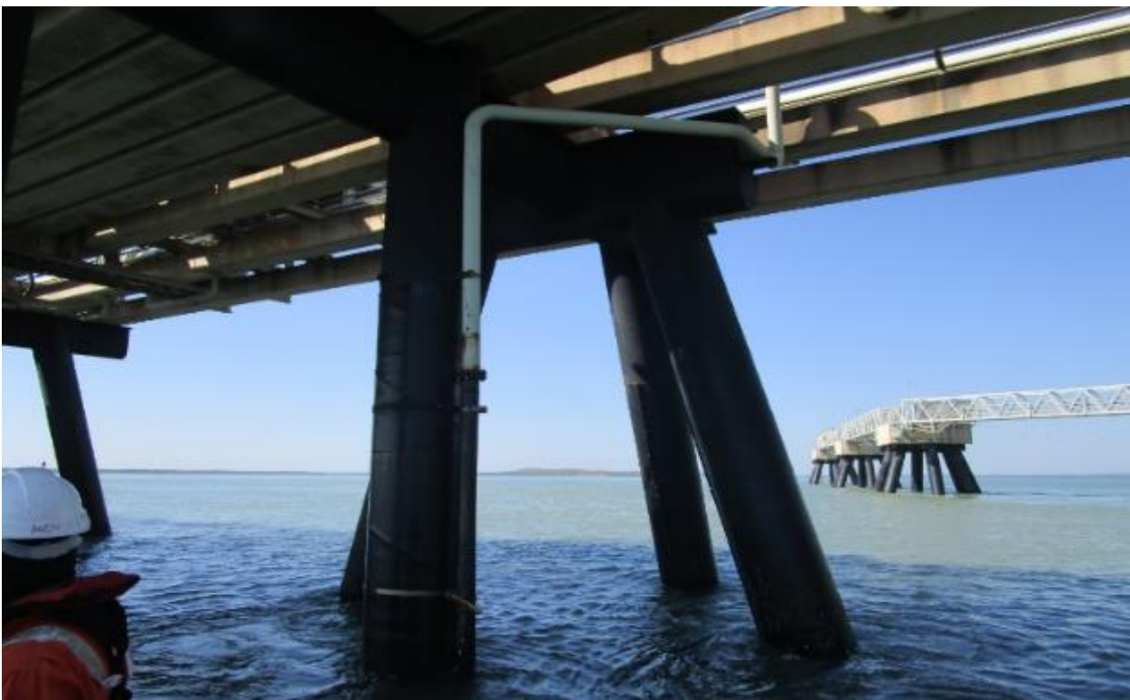
Figure 2-3 DLNG jetty outfall pipe secured to pylon
