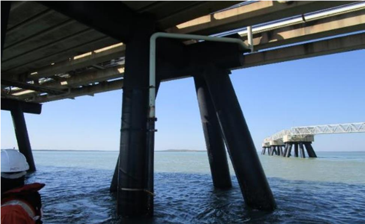
Figure 3-3 DLNG jetty outfall pipe (Secured to Pylon)
