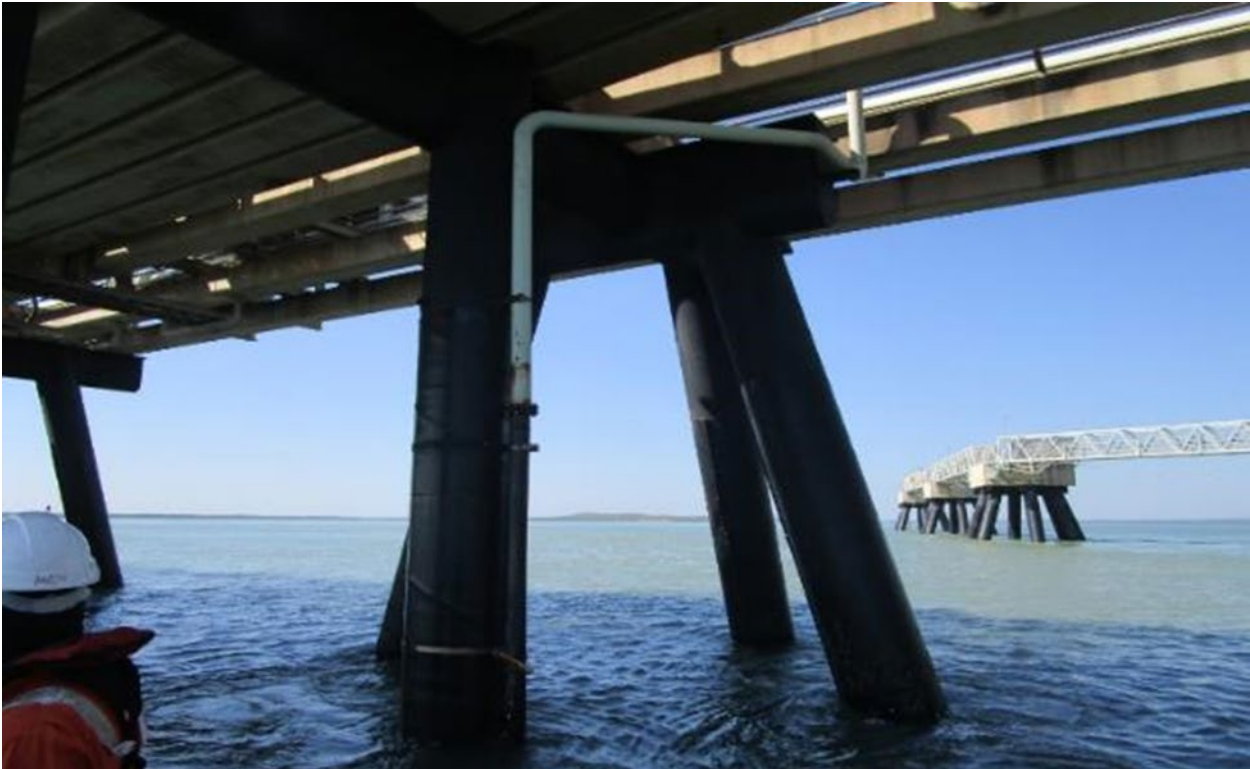
Figure 3-3 DLNG jetty outfall pipe (Secured to Pylon)
