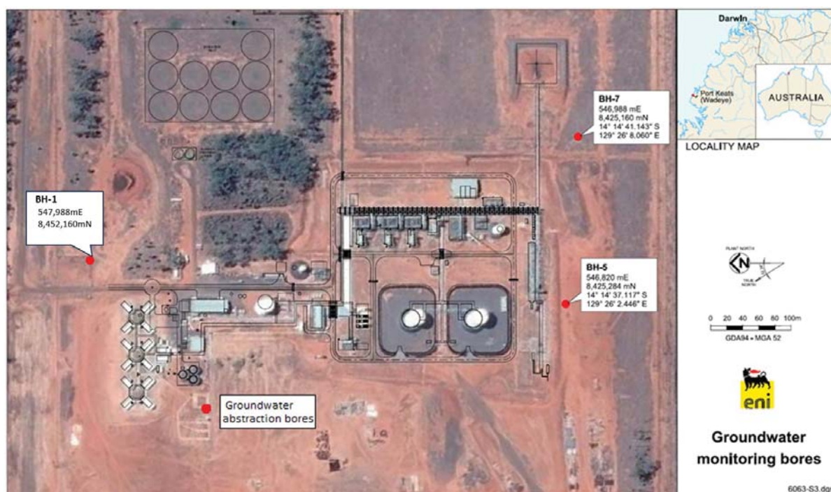
Figure 8.1: Groundwater abstraction and monitoring bores
