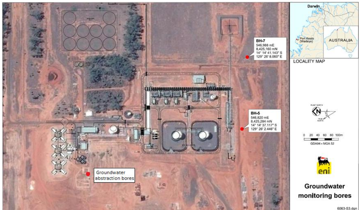
Figure 8.1: Groundwater abstraction and monitoring bores
