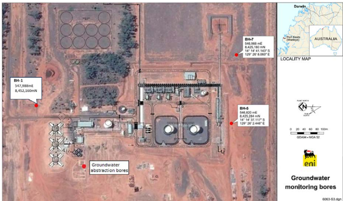
Figure 8.1: Groundwater abstraction and monitoring bores
