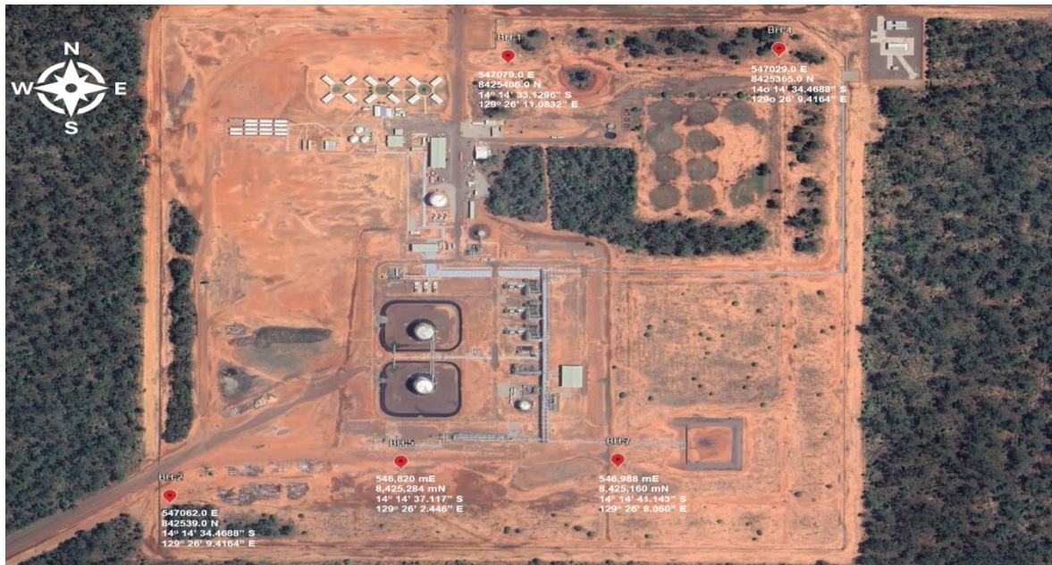
Figure 9-1: Groundwater abstraction and monitoring bores
