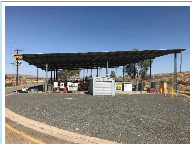
Photo 7 - Hazardous Waste Compound
