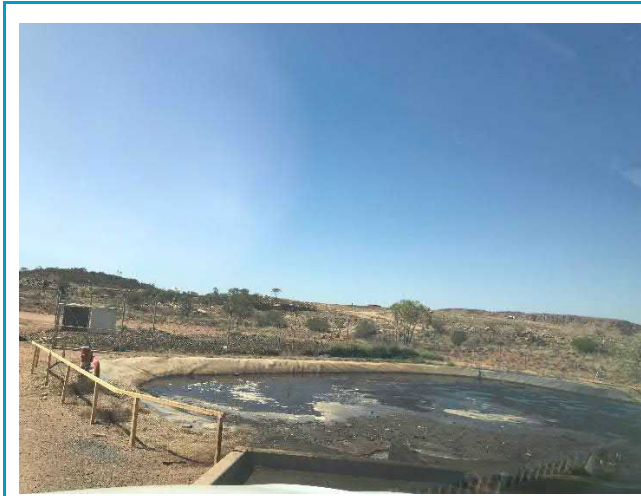
Photo 8 – Oily water storage pond
