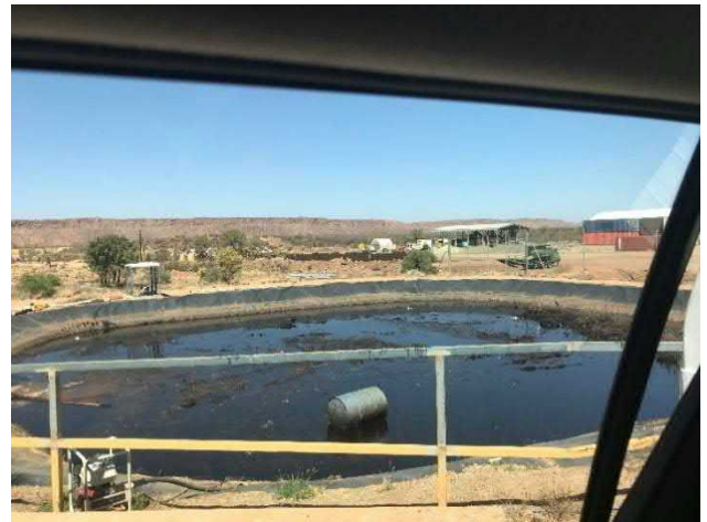
Photo 9 – Oily water storage pond
