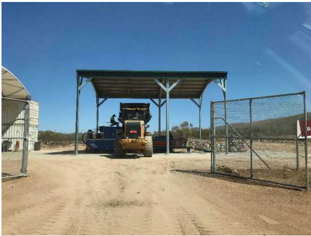
Photo 11 – Cardboard compacting facility
