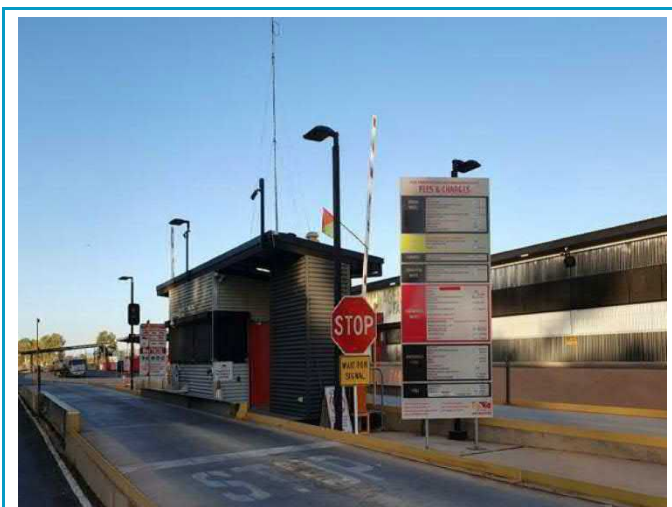
Photo 1 – RWMF Entrance and Weighbridge
