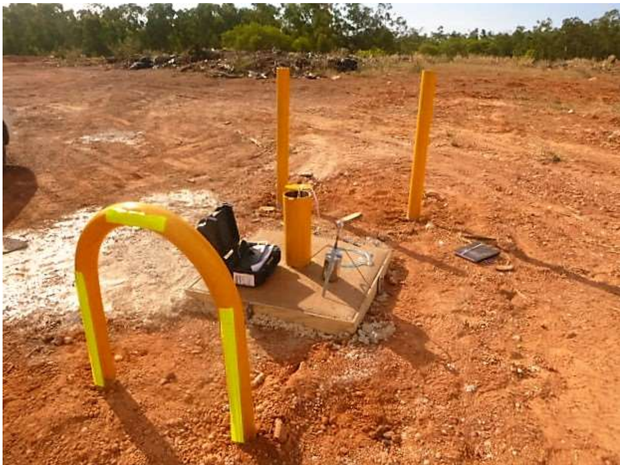
Figure 5: Landfill Gas Monitoring - Gove Peninsula Waste Management Facility
