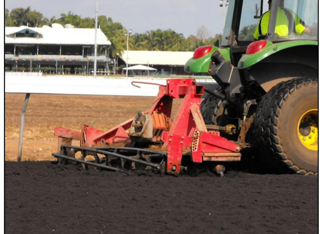
Photo 5: Tilling of track surface.
