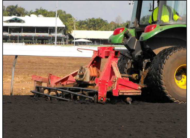
Photo 5: Tilling of track surface.
