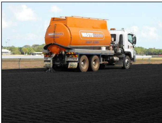
Photo 6: Application of oil to the track surface.
