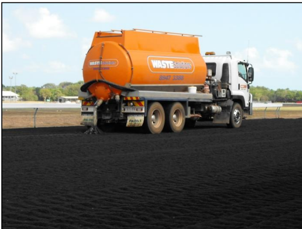
Photo 6: Application of oil to the track surface.
