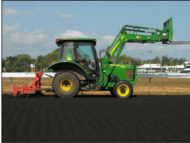
Photo 4: Tilling of track surface during oil application.
