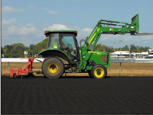
Photo 4: Tilling of track surface during oil application.
