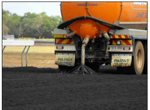
Photo 7: Application of oil to track surface.
