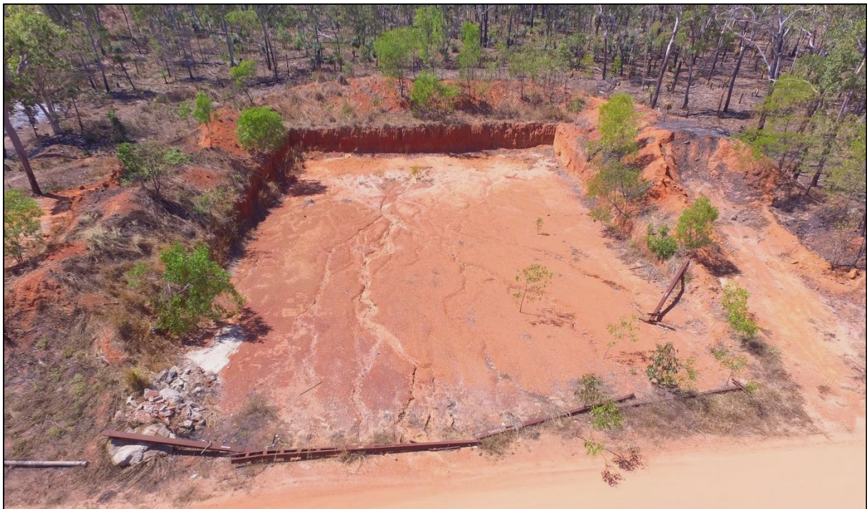
Figure 4.7 - Aerial photo of Cell 5 (29/08/2019)
