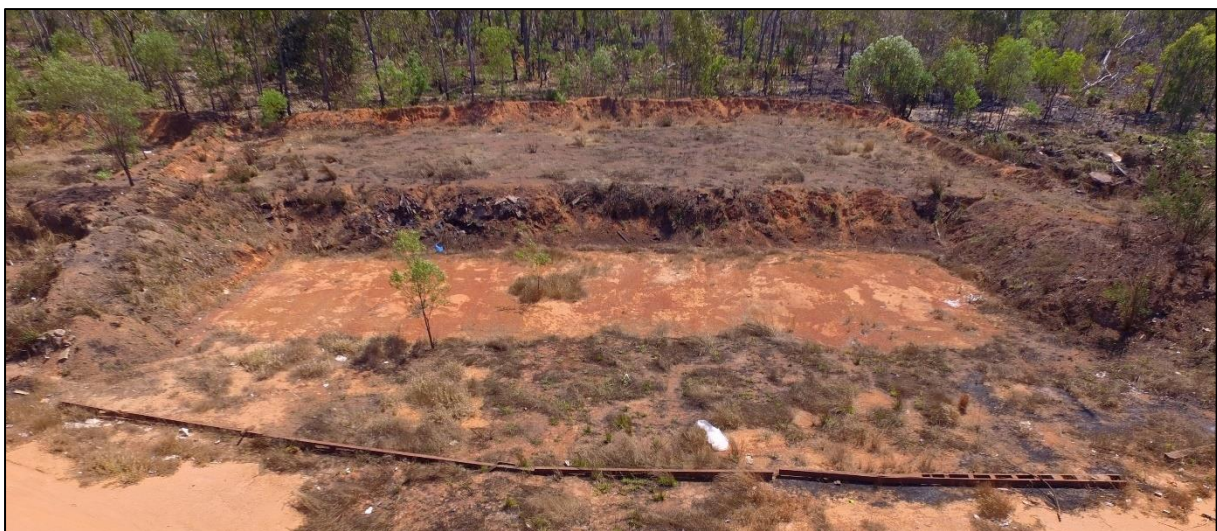
Figure 4.5 - Aerial photo of Cell 3 (29/08/2019)
