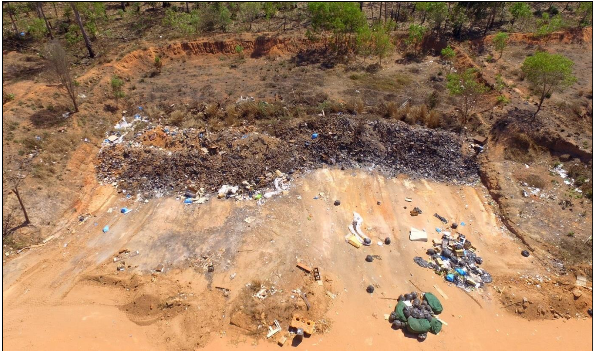
Figure 4.4 - Aerial photo of Cell 2 (29/08/2019)
