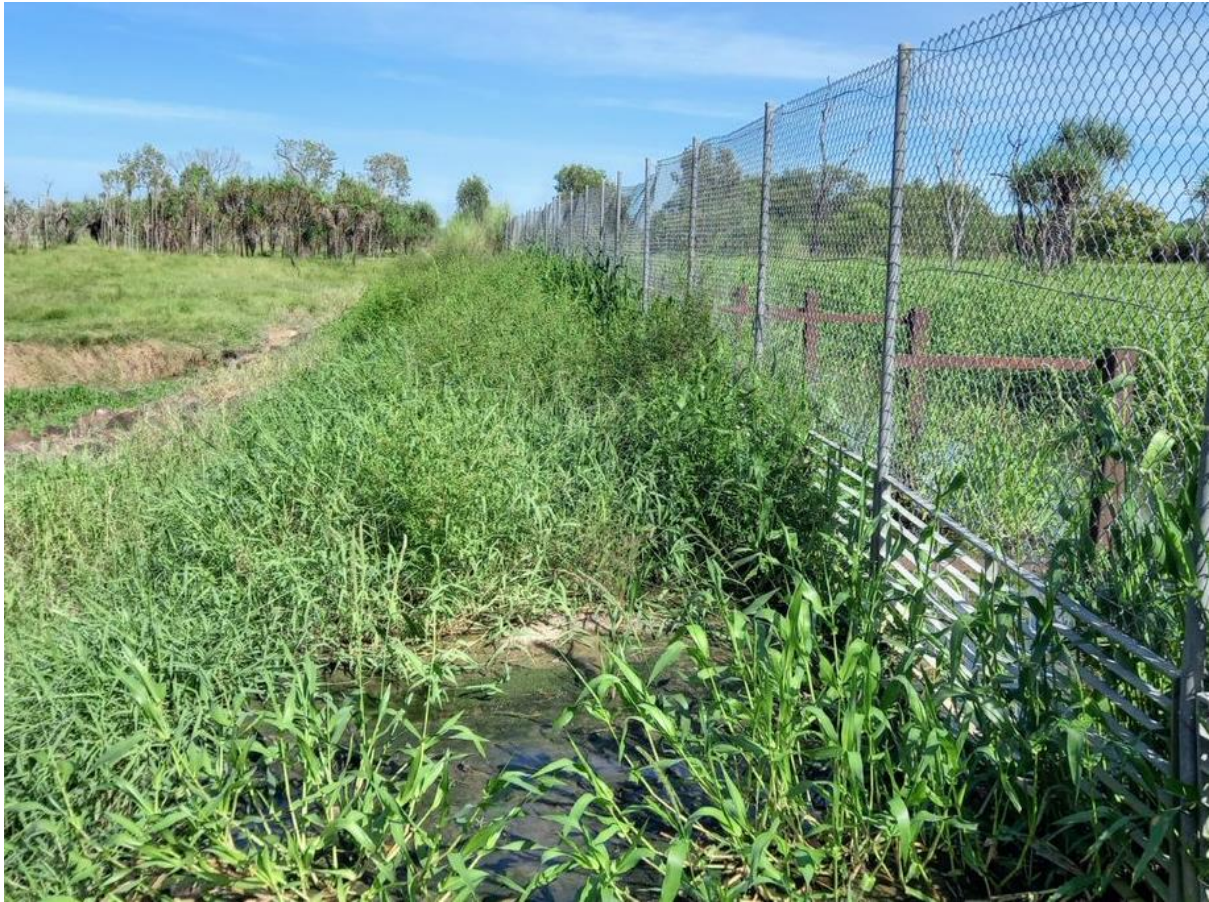
Figure 5 - End of wet season vegetation growth along the spillway
