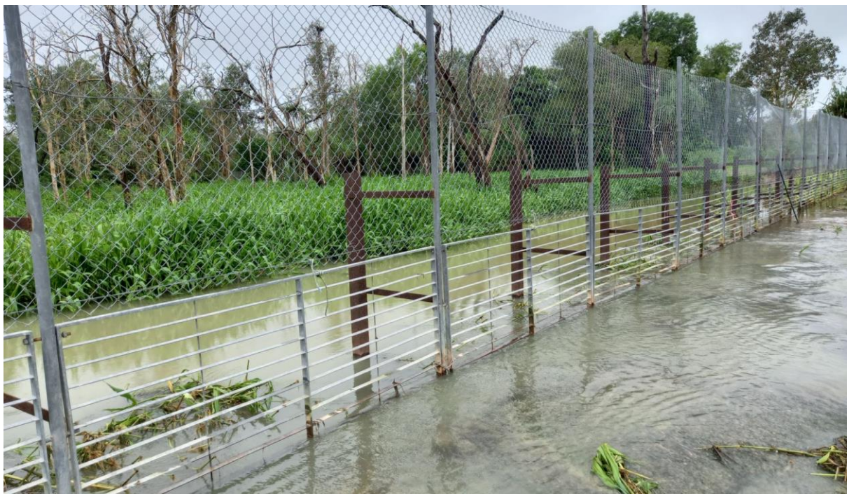
Figure 1 - Spillway and boundary fence
