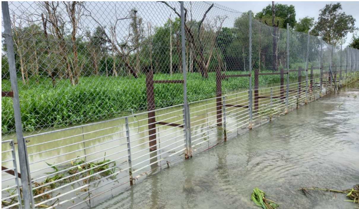
Figure 1 - Spillway and boundary fence
