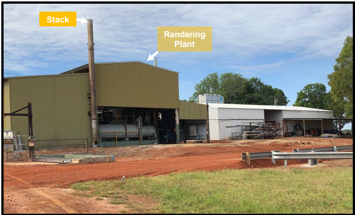
Figure 1.2 – Location of wastewater ponds and discharge stack from the dryer
