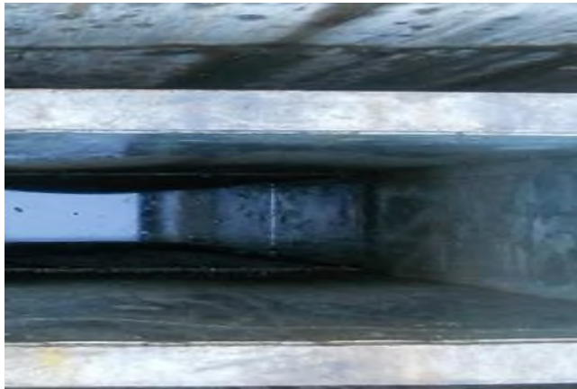
A view of unit A after being cleaned
