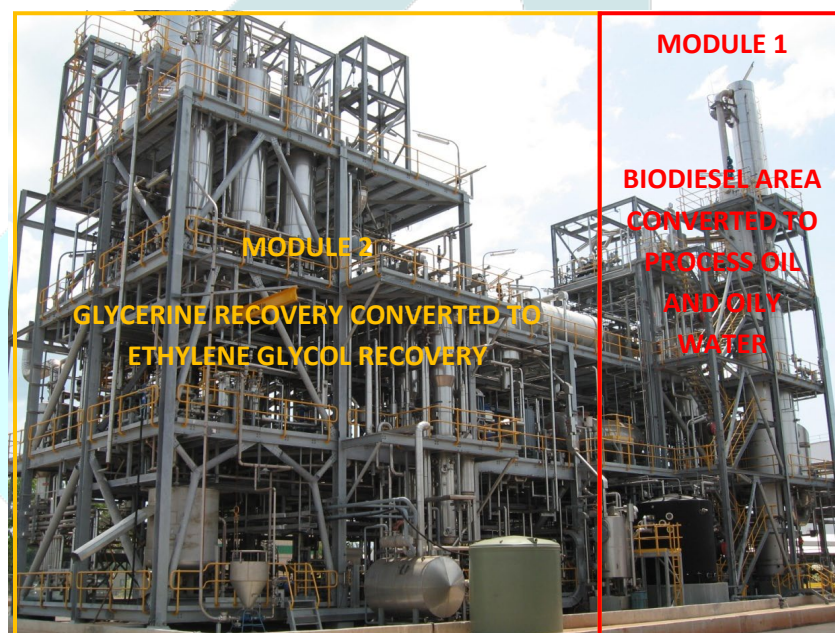
Figure 3: Existing Biodiesel Facility and Conversion to Oil and Glycol Treatment
