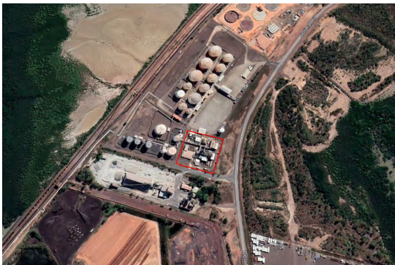
Figure 2 Darwin Liquid Waste Treatment Facility Close-up
