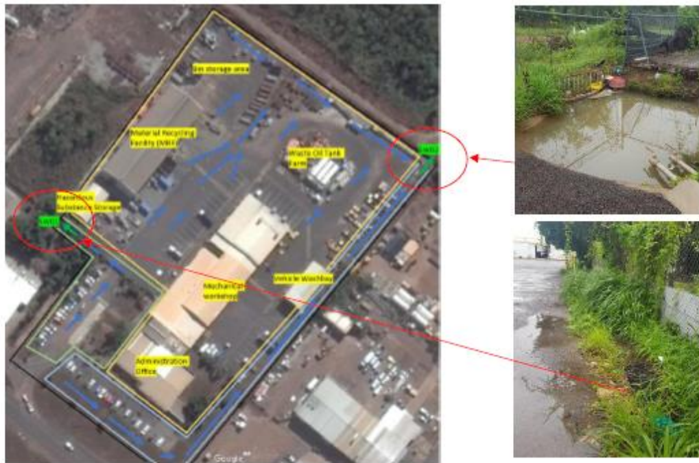
Figure 4-1 Location of Stormwater Sampling Locations – Holtze Facility
