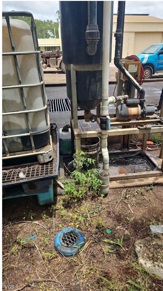
Figure 1-1 Vertical Gravity Separator (February 2024)
