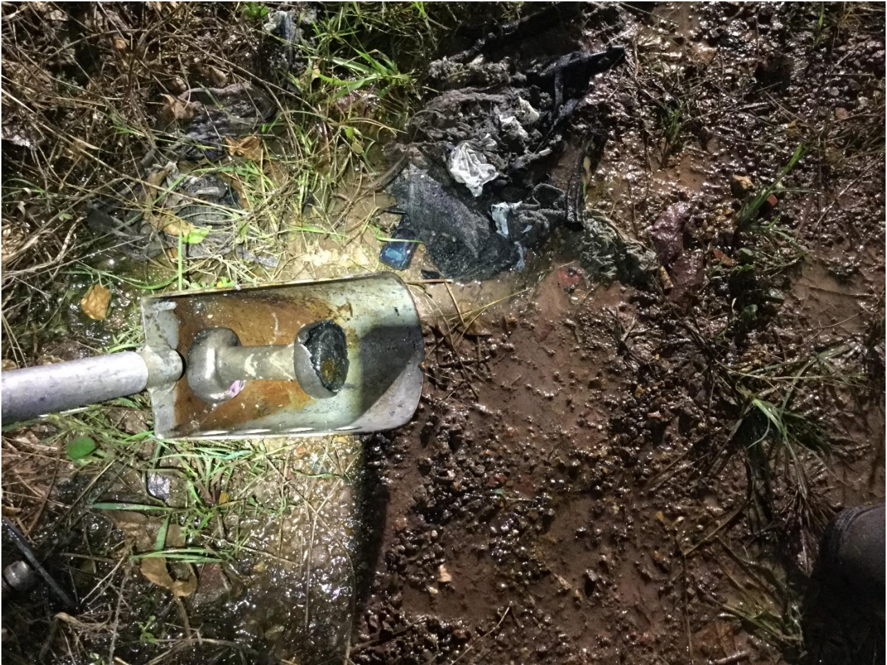
Appendix B – Photograph of some of the foreign matter found in the sewer network.
