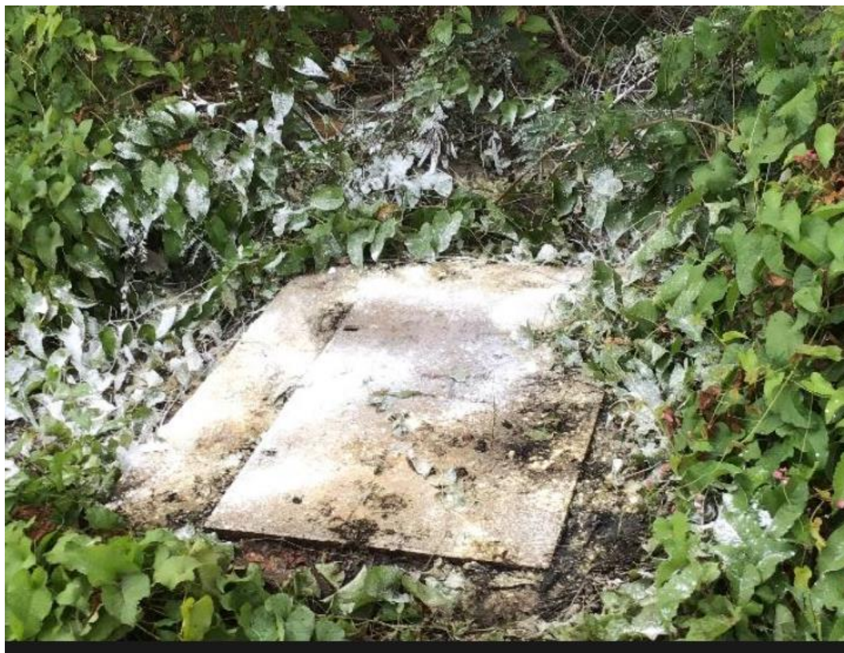
Photo 1 – Manhole (post cleanup)
