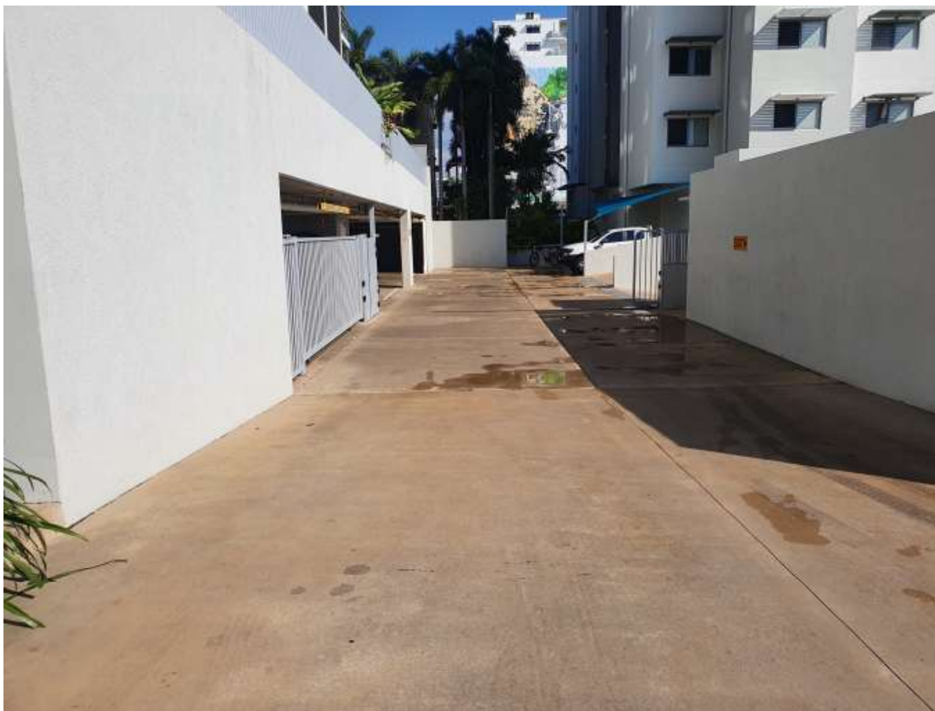
Photo 2 – Carpark driveway (post cleanup)
