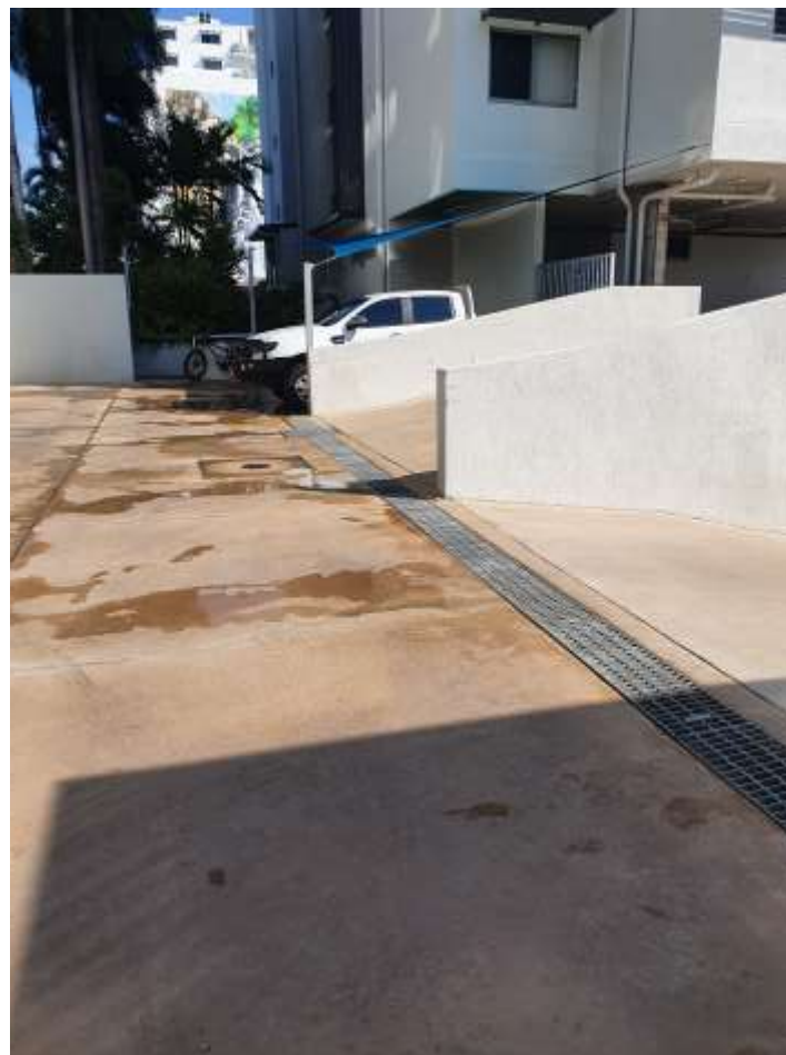
Photo 3 – Stormwater Drain (post cleanup)
