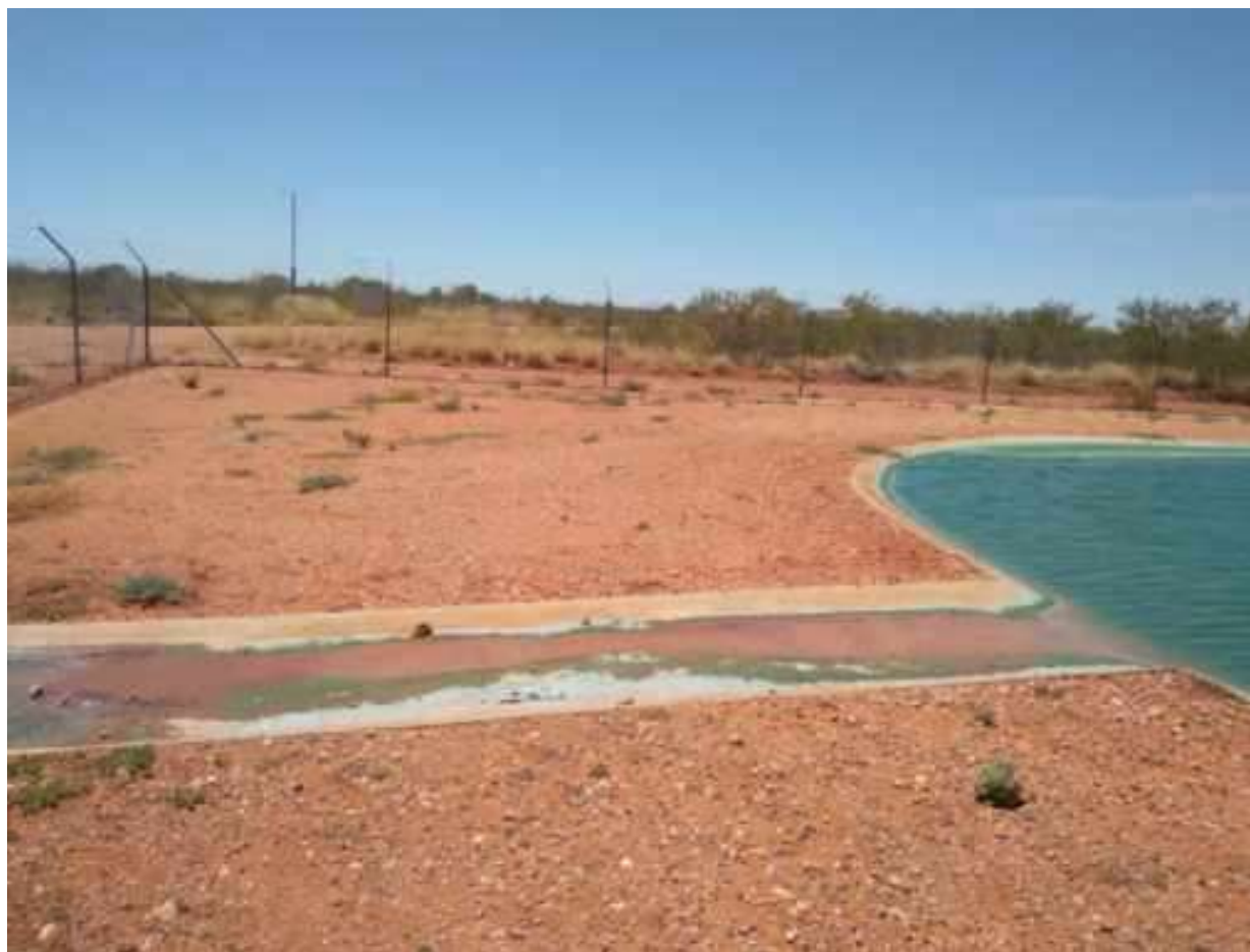
Figure 2 – Emergency overflow channel
