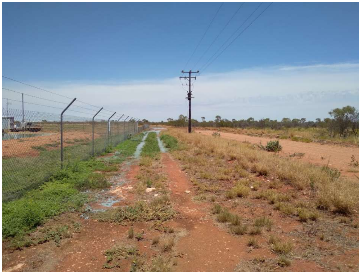
Figure 3 – Overflow site facing towards pooling
