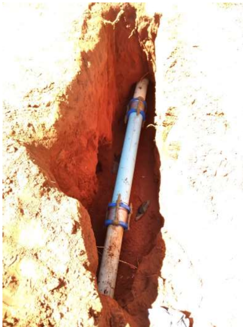
Photo 4 – Excavation with finished repair
