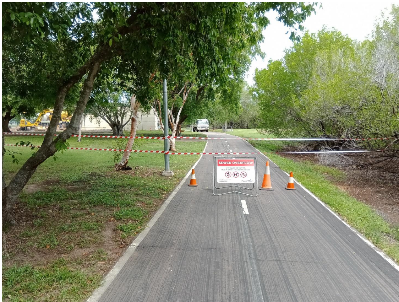
Figure 1. Warning signage erected, looking NNW along pathway
