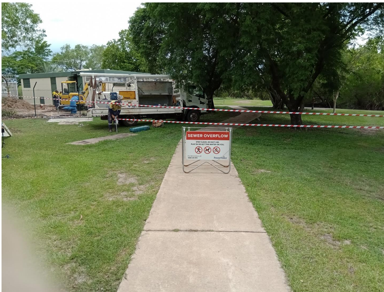
Figure 3. Warning signage erected, looking NE, from southern side of sewage pumping station.
